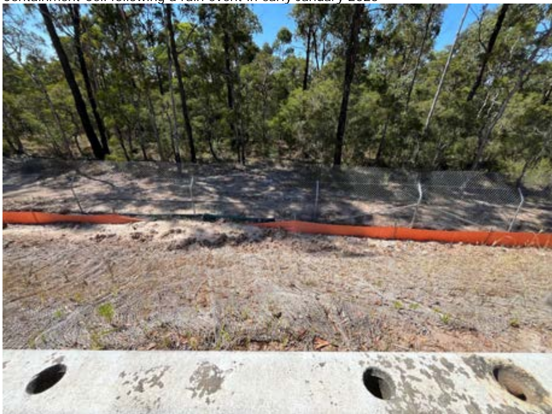
Photo 4: (January 2025): View of southern fauna fence and perimeter sediment fencing at the Containment Cell following a rain event in early January 2025
