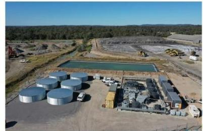
TWTP - Temporary Water Treatment Plant and LD03 treatment dam on 2/6/23. Some process problems experienced from mid-May to mid-July with high molybdenum. Media changeouts and other process changes were required. Now back in service.
