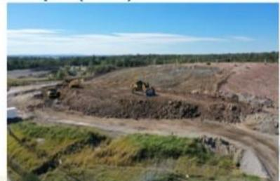
Stripping the clay cap at the CWS on 2/5/23, some of this material was used as fluffy layer in the cell
