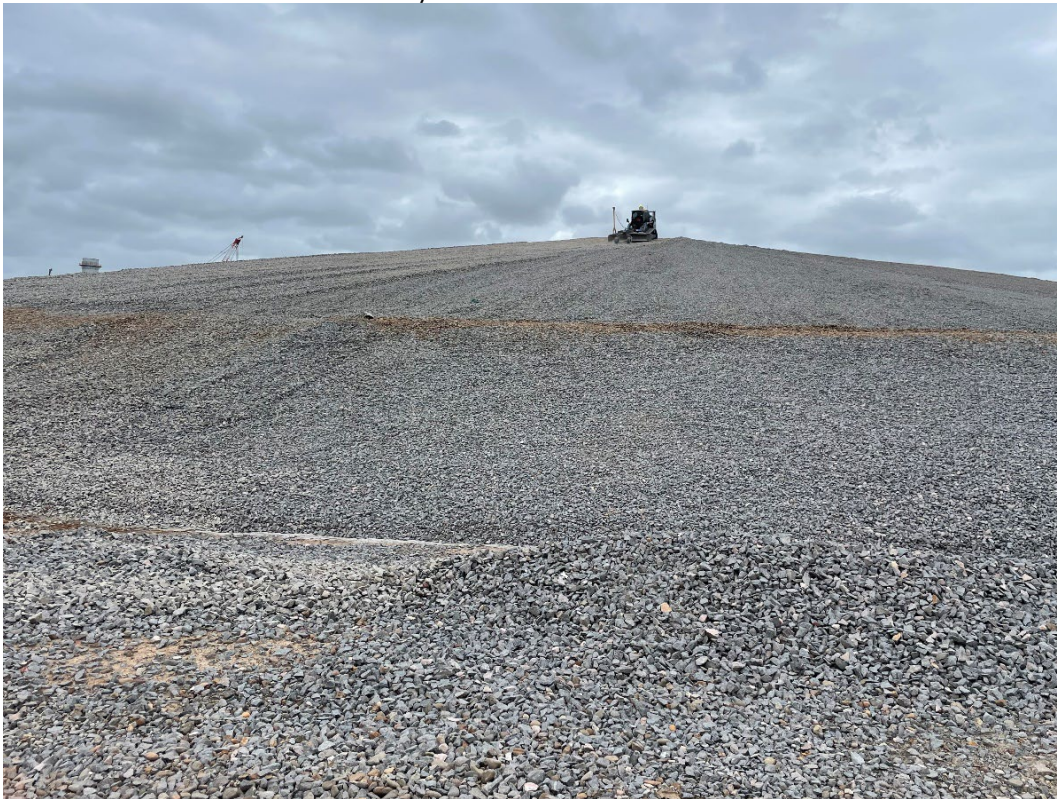
Photo 5: View looking over the placement of drainage aggregate sub-layer of the capping to part of the Containment cell in February 2024
