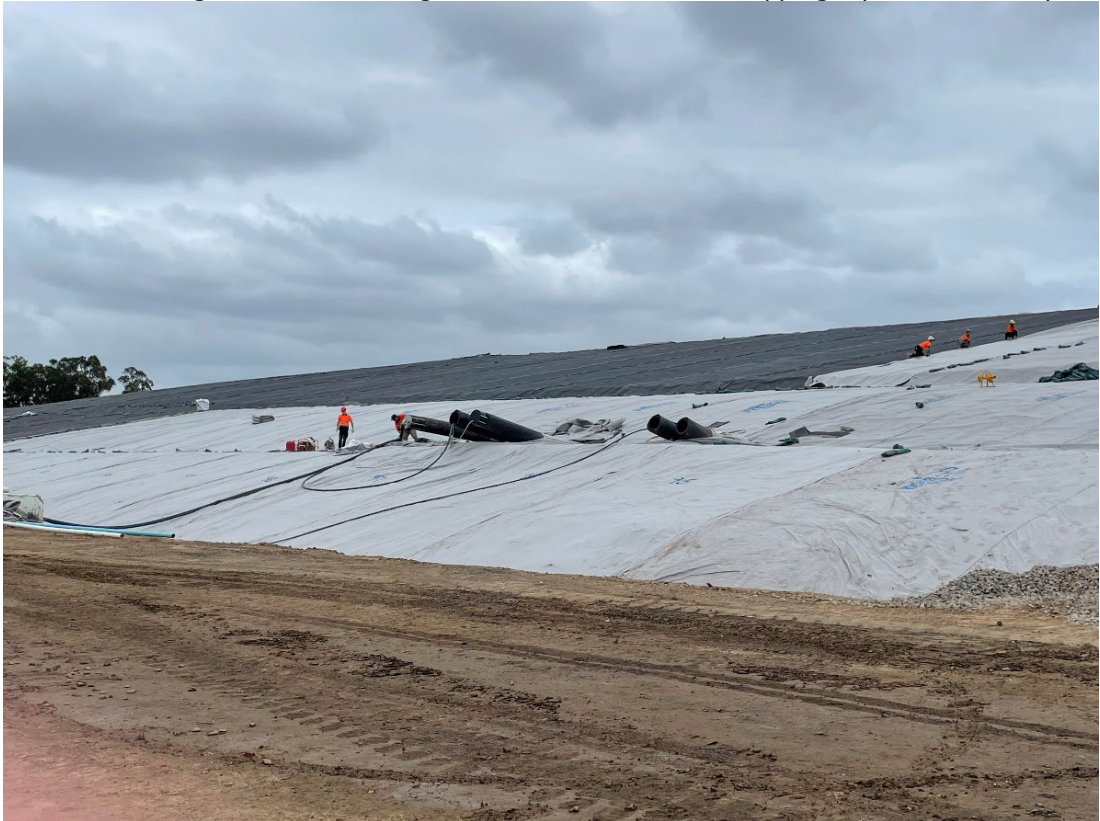
Photo 4: Looking north at the lining of the Containment Cell capping layers in February 2024.
