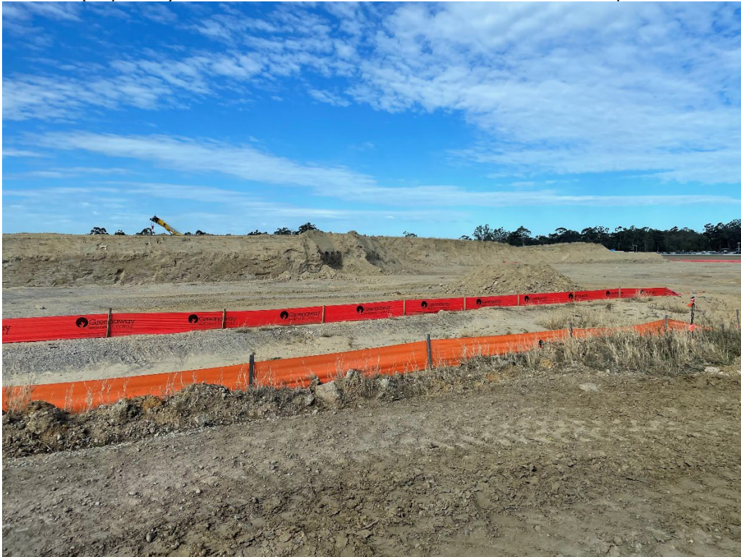
Photo 1: (July 2023) Erosion and sediment controls installed to soil stockpiles
