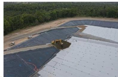
Start of waste transfer to the SE quadrant on Mon 13/2/23. This was the cement-stabilised pond sediments from the west surge pond. An initial pad of 'fluffy' layer material was placed at 1.7m thick using a 36T digger.
