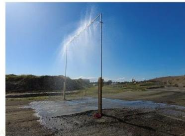
Water sprays being tested at the Capped Waste Stockpile as @ 28/4/23 prior to starting the removal of mixed smelter waste. The water helps to suppress any dust from the gypsum.
