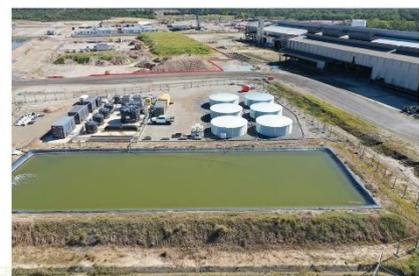
PHOTO: TWTP - Temporary Water Treatment Plant and LD03 treatment dam as @ 2/5/23. Note that both leachate from the ECC and the 7A sump is being treated. 27 hatches or 3.7ML of low fluoride leachate has now been treated.
