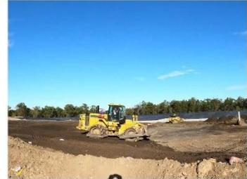
825 landfill compactor & D6 dozer working in the cell spreading & compacting waste on 12/4/23. Daracon and Hydro are keeping a close watch on the global density of the waste as measured by the total mass of waste transferred and the surveyed volume (currently it is 1.90 T/m<sup>3</sup> versus 1.60 T/m<sup>3</sup> minimum) as density affects volume.
