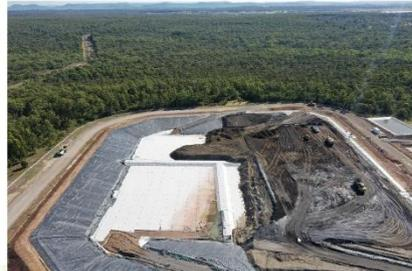
Aerial view of the cell as @ 12/4/23 - note that the SE and NE quadrants are being filled with waste and fluffy layer waste material has started to go into the NW quadrant. Leachate pipes connected and rain flap removed on the north saddleback.
