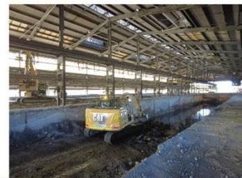
Process waste removal from 7A south tub as @ 28/4/23. Note water level in tub from rain water and ground water ingress. This water was around 40mg/L of fluoride and is treated at the TWTP. Waste has been removed & it has dropped to ~20mg/L of fluoride.
