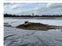
The dump trucks could then back out onto the pad and tip close to the edge where the dozer could spread the material. The dozer has GPS and is targeting a 1.7m thick layer that can be compacted and trimmed to 1.5m thick.
