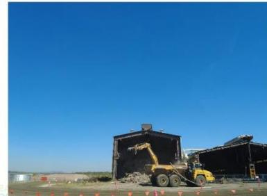
Removing demolition waste from 68C rubbish shed on 6/3/23. 20T excavator with grabs being used to load a 40T dump truck.
