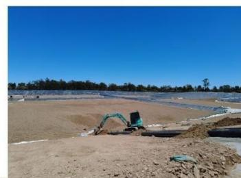
450mm diameter leachate riser pipes in the south sump with sand bedding layer installed and 300mm of soil confining layer being installed above the pipes – 13/12/22.
