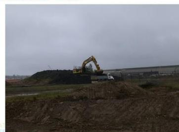
Anode butt fines being loaded into a 6-wheeler by 36T excavator fitted with load cells to cross-check weights with Hydro's weighbridge.
