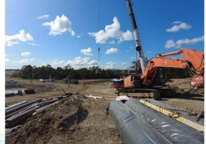
6T excavator being lifted into the south sump with the 300T crane for deployment of sand and drainage aggregate – 9/11/22.
