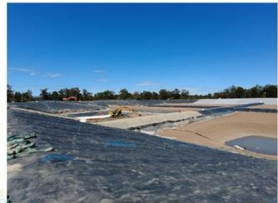
CRE PRO Preparation of subgrade on SE quadrant floor and eastern extremity of bund – 3/11/22.
