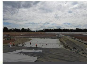
A34 separation geotextile deployed on floor ready for deployment of 300mm sand drainage layer – 11/11/22.
