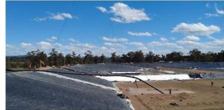
450mm diameter leachate riser pipes being installed in the north sump – 14/11/22.
