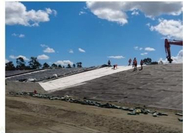
Deployment of primary GCL layer on eastern batter – 17/11/22.
