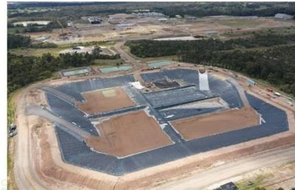
Aerial view of the cell – 18/10/22. A64 geotextile and drainage aggregate installed in three quadrants via the ramps, SE ramp started and work started on south sump.
