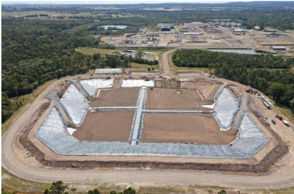
Aerial view of the cell – 14/12/22. Cell complete and ready to receive waste apart from completion of 1mm sacrificial geomembrane on eastern batter and completion of drainage aggregate in southern sump and base of the access ramps.
