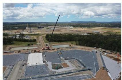
Sand and drainage aggregate deployment in the southern sump and GCL installation on the eastern batter – 9/11/22.
