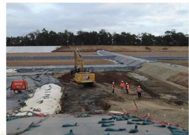
CRE PRO Subgrade preparation of floor in SE quadrant – 4/11/22. Unsuitable subgrade found due to presence of shale. Over-excavated by 200mm and replaced with suitable clay material.
