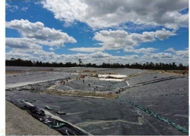
CRE PRO Installation of secondary liner patch (GCL & 2mm HDPE) – 26/10/22. Note that this is an additional liner – to make it the same as the north sump (3-layer sump).
