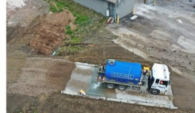
Filling of wheel wash by water cart. Note the use of blue dye to check for any carryover of contaminated water to nearby stormwater drains.
