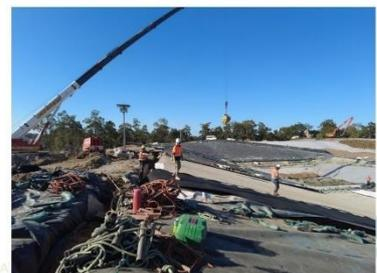
Subgrade prepared and secondary GCD deployment on eastern batter – 9/11/22. Note this was the last point of access into the cell for construction equipment. From here on the four access ramps must be used.
