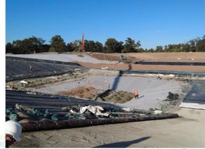
Placement of sand and drainage aggregate for the leak detection sump within the south sump – 9/11/22. Note adjacent floor has been lined with GCL and primary 2mm HDPE.
