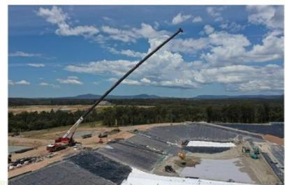
Deployment of sand on the floor of the SE quadrant using the kibble of the 300T crane – 12/11/22.
