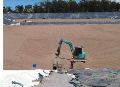
450mm diameter leachate riser pipes being installed in the south sump using an excavator – 8/12/22.
