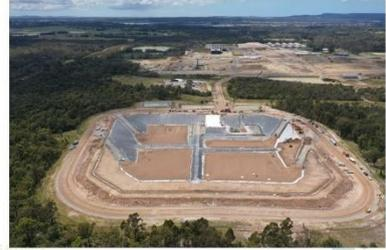
Overview of cell showing works in SE quadrant with 300T mobile crane in the background and soil confining layer deployment using a longreach excavator on the southern batter – 9/11/22.
