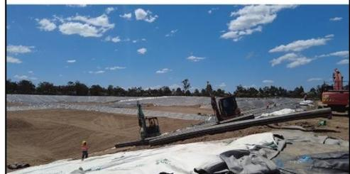
450mm diameter leachate riser pipes being installed in the south sump with two excavators – 9/12/22.
