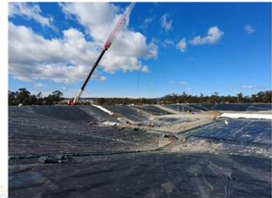
North sump repairs – deployment of GCL for secondary liner patch – 16/8/22.
