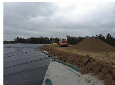
NW ramp - 150mm select fill layer being installed over the geogrid, followed by sub-base (150mm), base course (125mm) and wearing course (75mm) to complete the pavement. 800mm pavement layer above the primary liner suitable for 40T loaded dump trucks.
