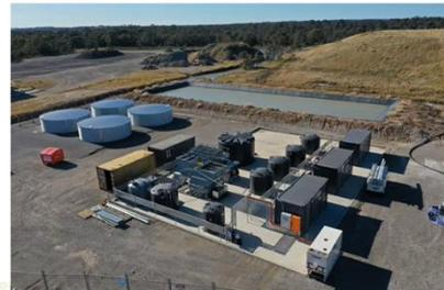
Temporary Water Treatment Plant on the 16/6/22 – dry commissioning completed, wet commissioning in progress with process commissioning to start in two weeks.
