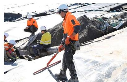
Arc testing of the existing HDPE secondary liner prior to patching on 15/8/22.
