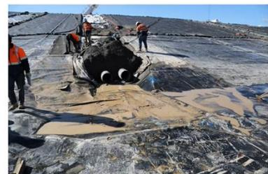
North sump repairs – leak detection pipes removed by crane and clean down of existing secondary liner - 15/8/22.
