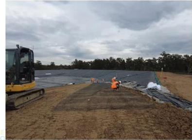
Soil confining layer installed on the NW access ramp and installing Tensar Triax Geogrid prior to installation of the four pavement layers – 12/8/22.
