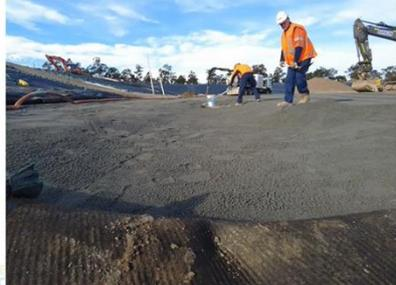
Preparation of the subgrade – NE quadrant floor prior to lining – 15/8/22
