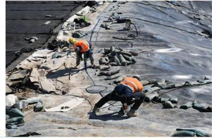
Secondary HDPE liner patch being extrusion welded to the existing secondary liner – 17/8/22. Small circles are patches at the T joints. Large patch is a DT sample.
