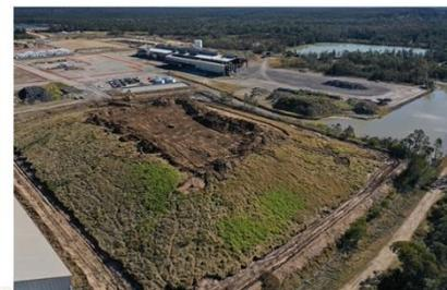
Stripping 0.5m of top soil from the Capped Waste Stockpile – 28/7/22.
