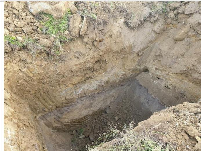
**Photograph 47:** AEC 33 Area East of the Clay Borrow Pit AECBP\_TP10. Foreign material observed.
