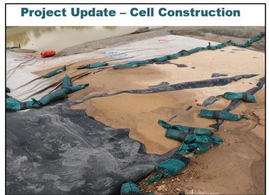
AW: That is a close up of the southern sump. We had a lot of problems with silt washing down from the top batter and also the stormwater bund that we built around the sump made its way into the sump. It was just unavoidable, the amount of rain we had. But they're cleaning that up now and we'll be getting back into it this week and next.
