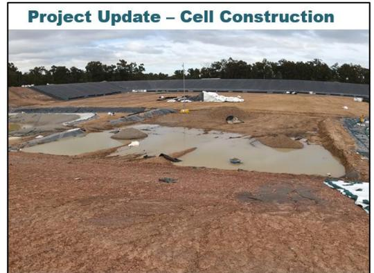
AW: This is a close up of the eastern ramp so this is the main access point that I mentioned. This was just after a rain event so they've been doing a lot of pumping of water for the last three weeks. That's the ramp in between the two sumps looking west.
