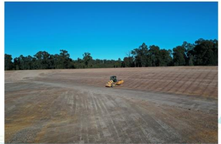
• ECC Rip & Recompact - Smooth Drum Rolling (20/7/21)
