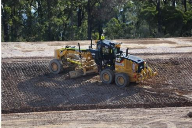
• ECC Rip & Recompact – Trimming Works (19/7/21)
