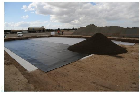
PK • Trial Pad to assess any damage to the HDPE caused by materials handling equipment and procedures (18/8/21)
