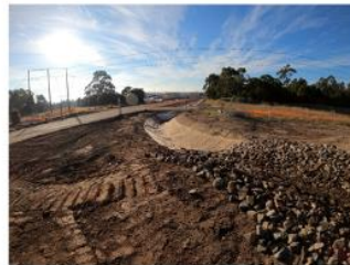
CREATING PROSPERITY FUTURES • ECC Works – Rip Rap outlet into Swale Drain 01 (6/7/21)
