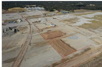
CRP PROSPERITY FUTURE • Leachate drainage aggregate stockpiles (21/6/21)
