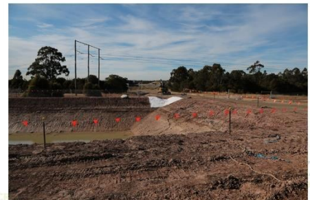
PRC • ECC Works – Sed Basin 1 Rip Rap Outlet (6/7/21)
