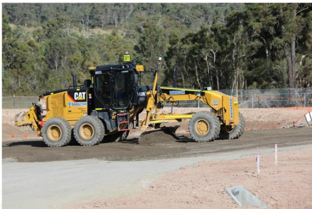
PRC • ECC Works – Grader trimming the sub-base layer on the ECC perimeter road (19/7/21)
