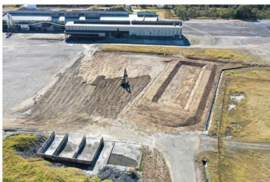
CRP PROSPERITY FUTURE • AEC2 – construction of Leachate Buffer Storage Pond and level pad for TWTP concrete slab adjacent to the Capped Waste Stockpile (5/7/21)
