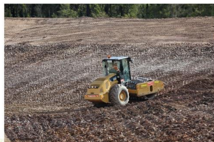
CREATING PROSPERITY FUTURES • ECC Rip & Recompact – Compaction Works (19/7/21)
