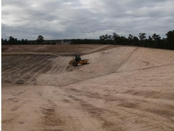
• ECC Rip & Recompact – Smooth Drum Rolling (21/7/21)
