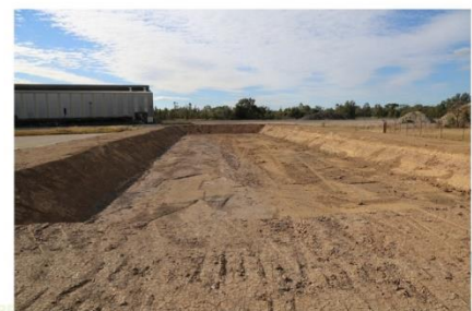
CREATING PROSPERITY FUTURES • ECC Works – Leachate Buffer Storage Pond (19/7/21)
