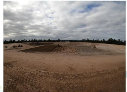
• ECC Rip & Recompaction of Base (21/7/21)
