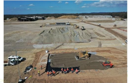
• Trial Pad to assess any damage to the HDPE caused by materials handling equipment and procedures (18/8/21)
