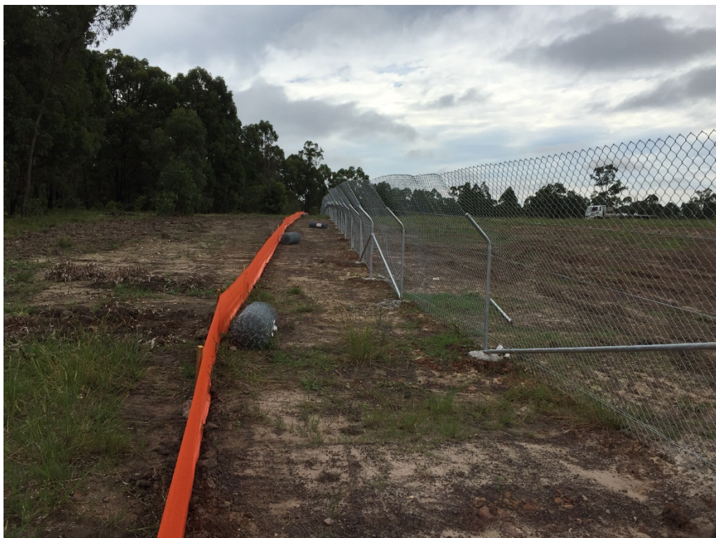
Photo 2: View looking north along the western boundary to the Containment Cell area, showing the sediment fencing and the fauna proof fencing.
