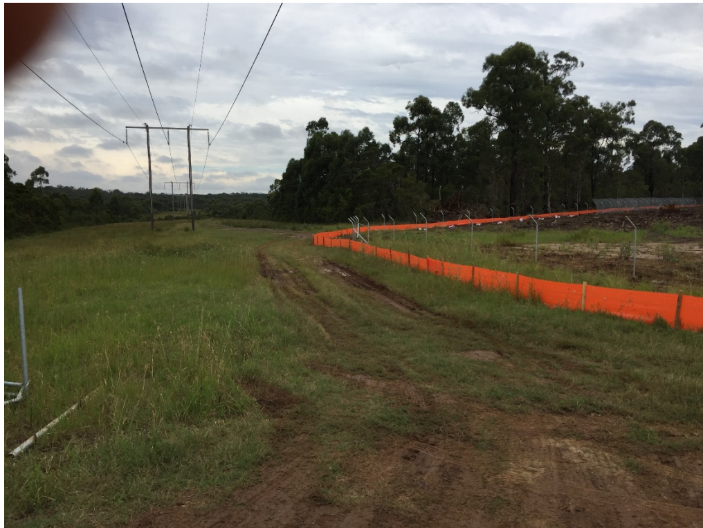
Photo 1: View looking west along the southern boundary to the Containment Cell area, showing the sediment fencing (in orange) and part of the fauna proof fencing.
