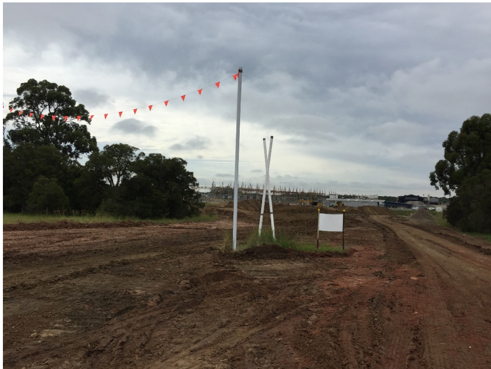
Photo 3: View looking east from the Containment Cell area towards the Smelter showing safety controls for vehicles passing below the overhead powerlines.
