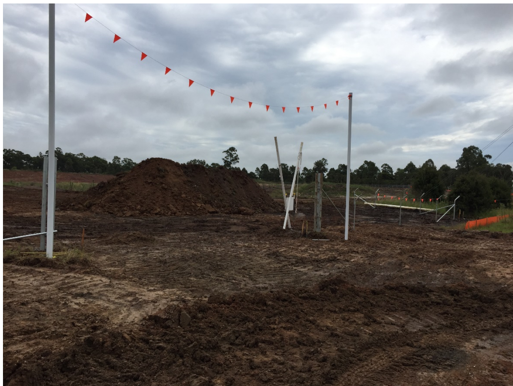
Photo 4: View looking north along the eastern boundary to the Containment Cell area showing additional safety controls for vehicles passing below the overhead powerlines.
