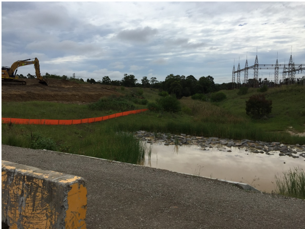
Photo 5: View looking north from the existing crossing of the unnamed creek showing sediment fencing and earthworks that were underway are shown in the left (west) of the photo).
