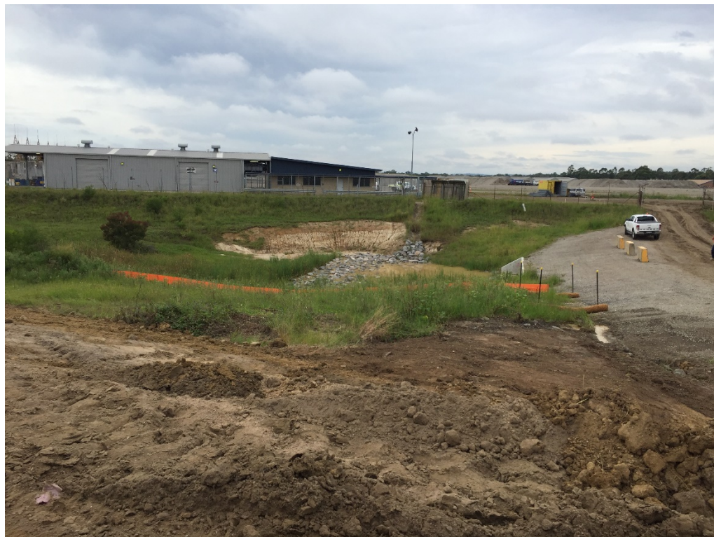
Photo 6: View looking east from the Containment Cell area towards the Smelter showing sediment controls.
