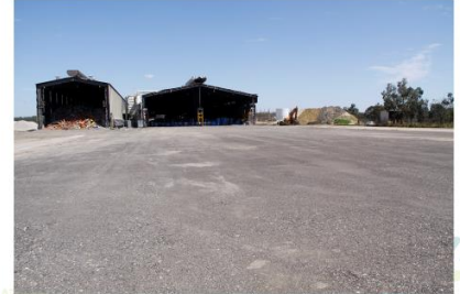
Milled asphalt was used as fill material at the Anode Bake Furnace. Material was graded and compacted to create a free draining surface
