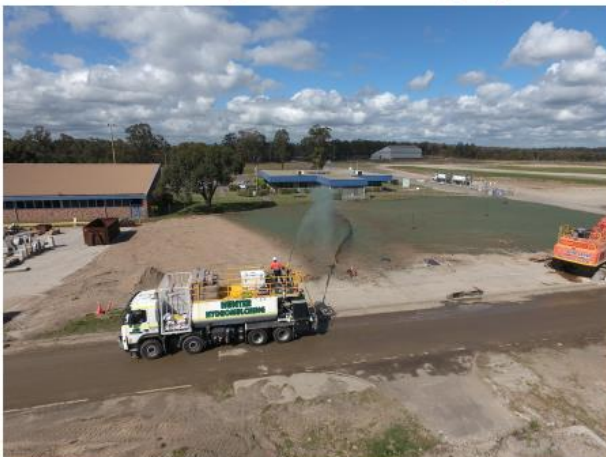
Seeding & Hydromulching of 25A Building Footprint to Minimise Dust (29/9/20)
