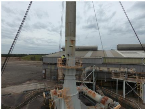
Demolition of the 7B bypass stack – oxy lancing the birds mouth cut (30/9/20)
