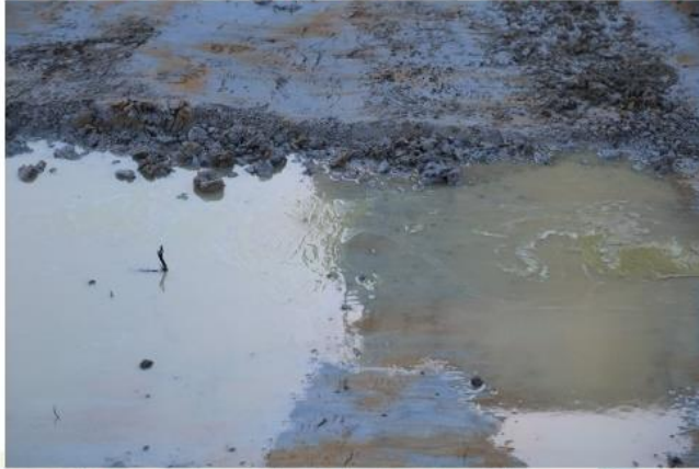
Digging up contaminated soil at the location of the rodding presses & cable trenches – note oily residue on surface of water (1/7/20)
