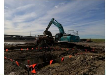
Digging out an old oil separator and grease pit adjacent to the mechanics pit found in 26B ATC Building (3/8/20)
