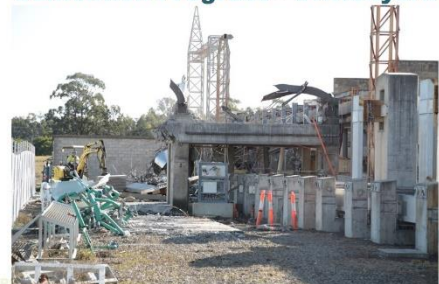
Switchyard demolition – Line 3 last bay & busbar (26/6/20)
