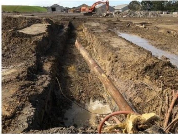
Removal of redundant 30A fuel oil & services trench (11/8/20)
