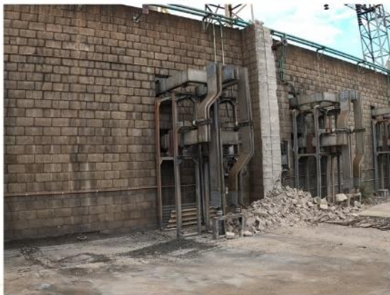
Asbestos packers on Line 1 busbar supports(10/7/20)
