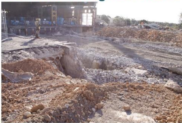
CRP PROSPERO FUTURES Demolition of Southern Tub Wall & Refractory Backfill (29/6/20)
