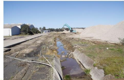
Removal of stormwater drain & culverts along main road (21/7/20)
