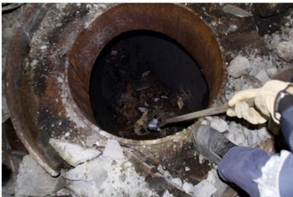
Removal of 7A Ring Main Brick Lining for Sampling & Testing (23/7/20)
