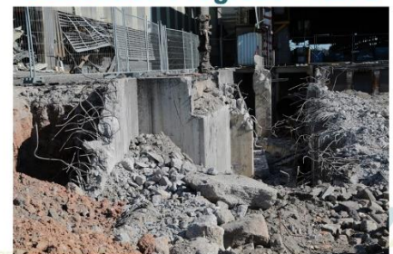
CRP PROSPERO FUTURES Demolition of Southern Tub Wall, Building Columns & Retaining Wall (1/7/20)
