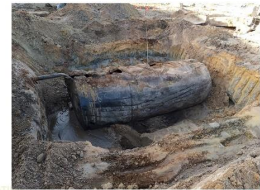
UST for petrol at 26B ATC Building – tested with a PID by Ramboll. Volatiles as measured by LEL reading were non-detect proving that it was safe to allow removal. (3/8/20)
