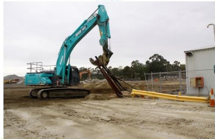
Removal of cables at former 30A Fuel Oil Bund (12/8/20)
