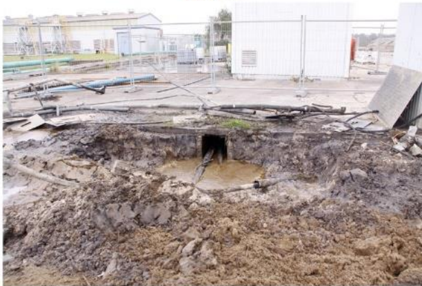
Demolition of 30 A Fuel Oil Bund with 37A sewer pump station in the background (10/8/20)
