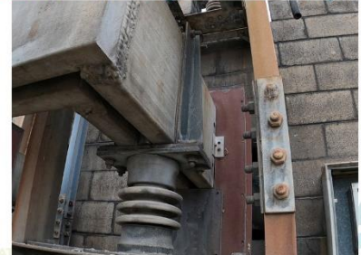
Asbestos packers on Line 1 busbar supports(10/7/20)
