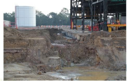
Digging up contaminated soil at the location of the cable trench between 7A & 8A (2/7/20)
