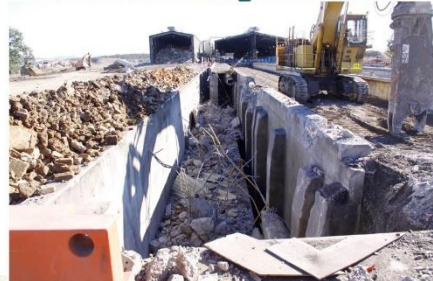
PROGRESS FUTURES Demolition of Building Columns, Removal of Ring Main, Flooring & Structural Steel (19/6/20)
