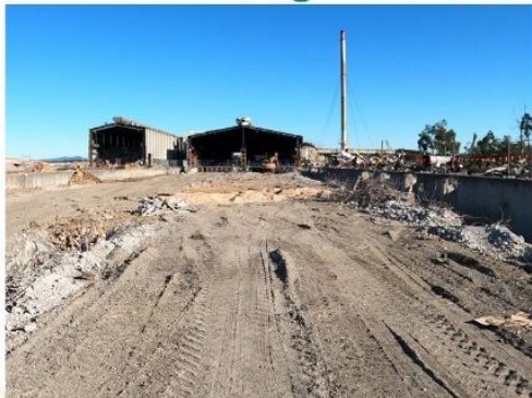
ABF2 – north tub – most tub walls removed and voids backfilled (25/6/20)
