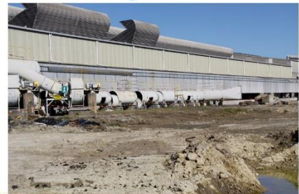
7A Bypass Duct & Fan demolition (4/8/20)
