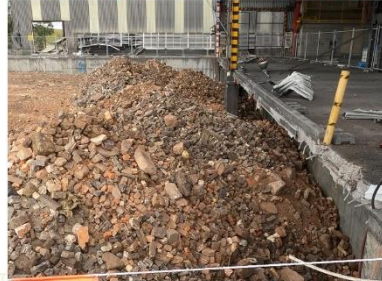
ABF2 – Refractory backfill at western end (10/7/20)
