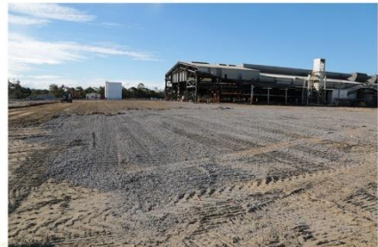
Backfilled and graded excavation at former rodding presses & cable trenches (9/7/20)
