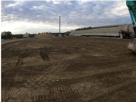
Backfilled and graded excavation at the location of the 8C / 96A area with the contaminated soil stockpile in the background (10/7/20)
