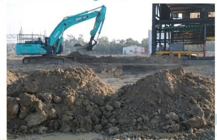
Digging up contaminated soil at the location of the rodding presses & cable trenches (30/6/20)
