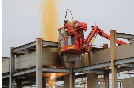
Switchyard demolition – lancing of busbars (14/8/20)
