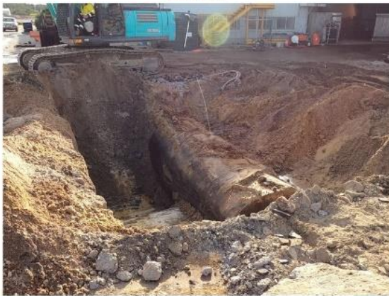
Underground storage tank (UST) for petrol found at 26B area (3/8/20)
