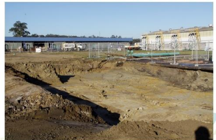
Further removal of contaminated soil from the 30A Fuel Oil Bund (13/8/20)
