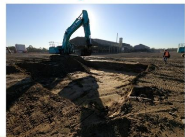
Thimble press hydraulic room footprint dig following some test pits that showed high readings for hydrocarbons (13/8/20)
