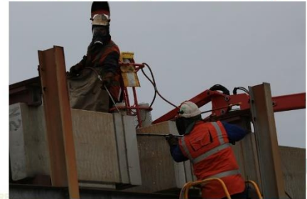
Switchyard demolition – lancing of busbars (14/8/20)
