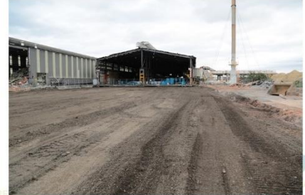
ABF2 Milled Asphalt Backfill (17/7/20)
