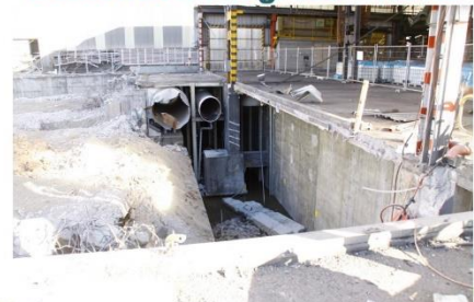
CRP PROSPERO FUTURES Demolition of Western End Crossover & Ring Main (29/6/20)
