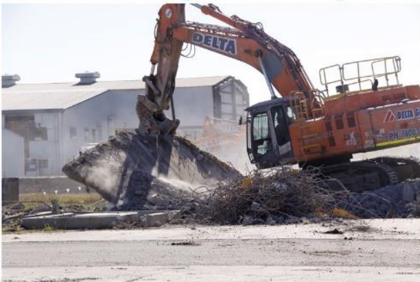
Removal of Cooling Tower CT4 Base (21/7/20)
