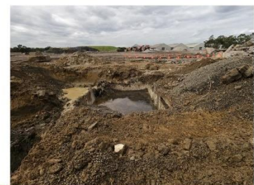
Mechanics pit found in 26B ATC Building (31/7/20)
