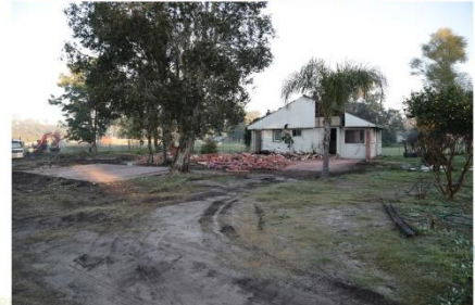
Aluminium cladding removed, revealing asbestos cement cladding, which required removal prior to commencement of demolition of house at 5 McLeod Rd (30/6/20)
