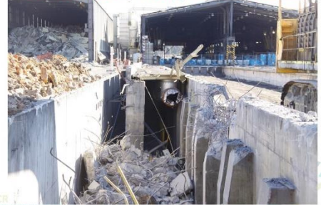
CR PROSPERIOUS FUTURES Demolition of Building Columns, Removal of Ring Main, Flooring & Structural Steel (19/6/20)
