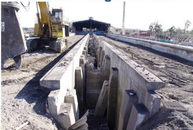
CR PROSPERIOUS FUTURES Central Void Between N & S Tubs Showing Centre Columns & Grid N Pile Caps (19/6/20)
