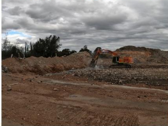
ABF2 Eastern End – pulveriser breaking down retaining wall (8/7/20)
