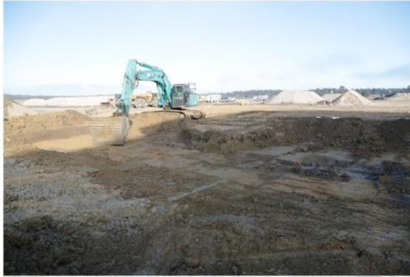
Digging up contaminated soil at the location of the rodding presses & cable trenches (30/6/20)
