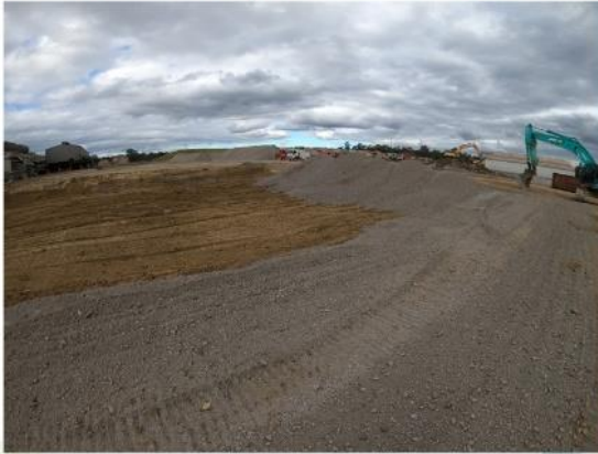
Backfilling of the excavated rodding press & cable trench area following successful remediation (8/7/20)
