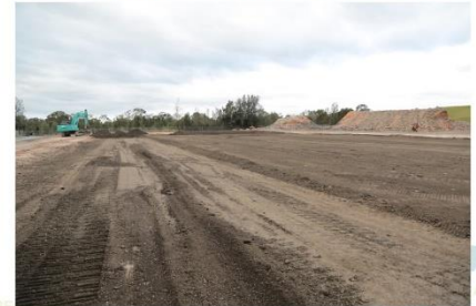
ABF2 Milled Asphalt Backfill (17/7/20)
