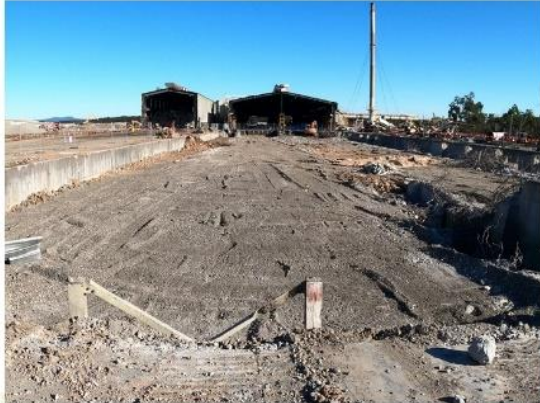
ABF2 – south tub – most tub walls removed and voids backfilled (25/6/20)
