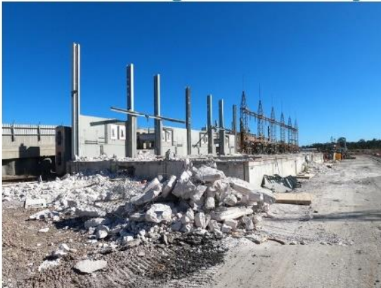
Switchyard demolition – 6A & 7A rectifier bays (5/8/20). Hebel concrete panels used for blast walls on these rectifier bays (&5B).
