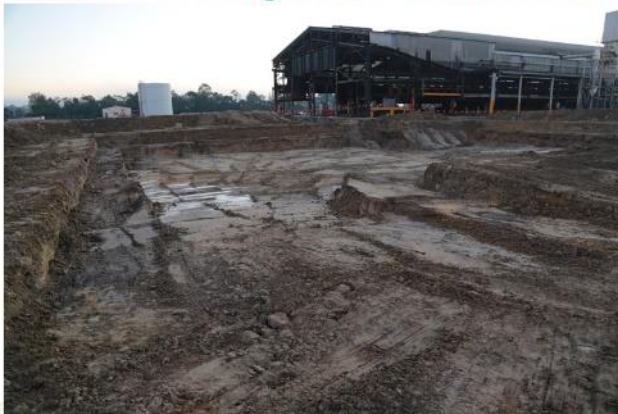
Further digging up of contaminated soil at the location of the rodding presses & cable trenches (2/7/20)
