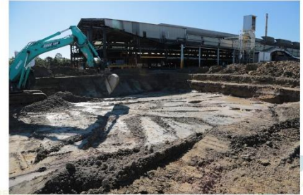
Digging up contaminated soil at the location of the rodding presses & cable trenches (1/7/20)
