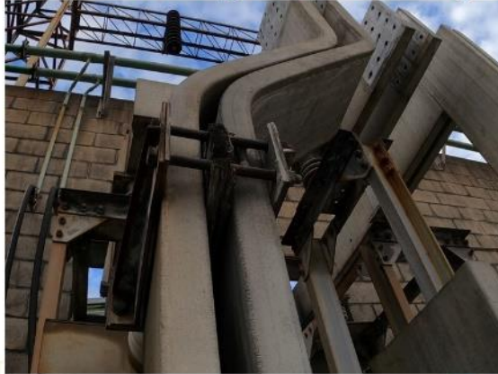
Asbestos packers on Line 1 busbar supports(10/7/20)
