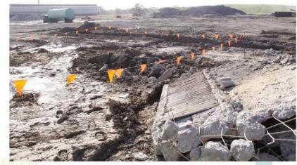
Footprint of former 26B ATC Building (31/7/20). Note corrugated iron cover over former oil separator and grease trap duct (which turned out to be asbestos).
