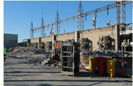
Switchyard demolition – Line 1 rectifier bays (1/7/20)
