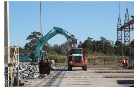
Switchyard demolition – removal of concrete debris (1/7/20)
