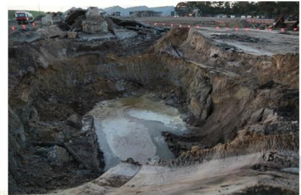
Footprint of former petrol UST – minimal contamination, excavated to remove any contaminated soil, sampled, tested and backfilled (4/8/20)
