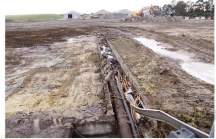
Redundant fuel oil & services trench south of 30A area (11/8/20)
