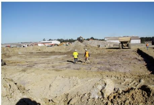
Digging up contaminated soil at the location of the rodding presses & cable trenches (30/6/20)
