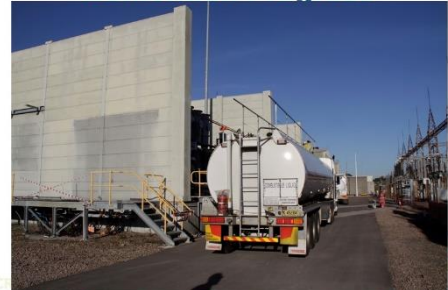
CREATING PROSPEROUS FUTURES Oil removal from 6A transformer to allow it to be scrapped (2/3/2020)
