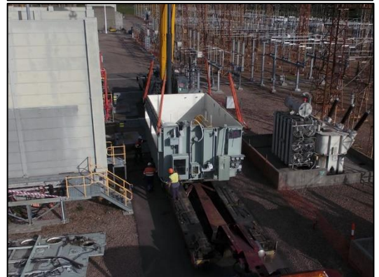
CREATING PROSPEROUS FUTURES Oil removal from 6A transformer to allow it to be scrapped (2/3/2020)
