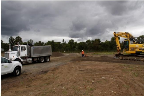
Remediation of the old Fire Training Ground (17/3/2020). Traces of PFAS found. Similar treatment as for PCB-contaminated soils. Sent to the SOLVE facility at Altona, Vic for heat treatment following EPA approval.
