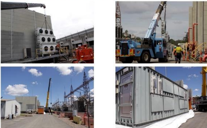
Removal of control rooms, A/C's, DC isolator switches and rectifiers for Trimet (Feb'20)
