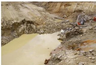
Removal of further oily water from butt tunnel excavation (3/12/19)
