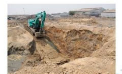
Final removal of concrete sump from butt tunnel (5/12/19)
