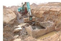
Final removal of concrete sump from butt tunnel (5/12/19)
