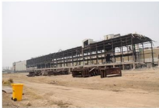
Line 3 Pot Shell Removal & Concrete Pulverising (9/12/19)
