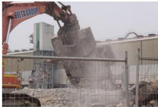
Line 3 Pot Shell Removal & Concrete Pulverising (9/12/19)
