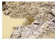
Butt tunnel excavation - free phasing of oil and oil-stained soil (3/12/19)
