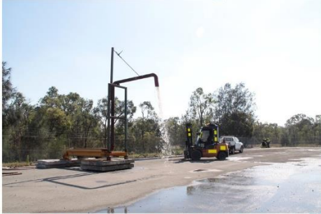
Setting up a standpipe at the East Surge Pond for dust suppression (4/12/19)
