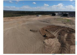
D5 dozer in operation to create a free-draining site
