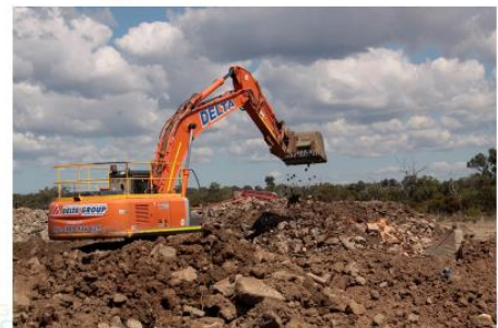
Sieving of Clay Borrow Pit stockpiles (20/9/19)
