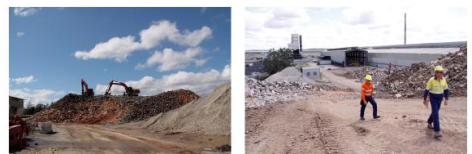
Refractory stockpile south of ABF2 – to be used for backfilling bake furnace tubs and basement voids once all SPLs has been removed and sent for recycling
