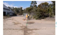
CREATING PROSPEROUS FUTURES Marking out pavements for milling of asphalt (20/9/19)
