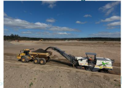
Milling of asphalt from roadways (9/10/19)
