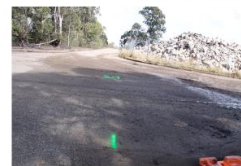
CREATING PROSPEROUS FUTURES Marking out pavements for milling of asphalt (20/9/19)
