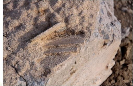
Bonded asbestos in underside of Line 2 basement slabs (22/3/2019)
