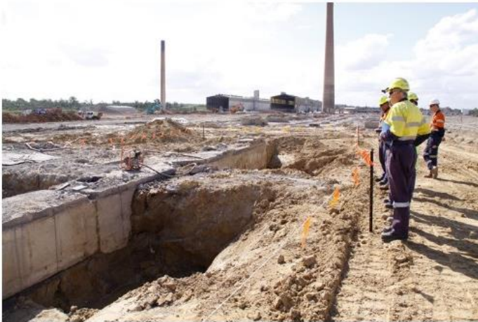
Line 1 fume duct culverts after saw cutting (10/4/2019)
