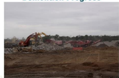
Concrete Crushing and Screening (7/3/2019)
