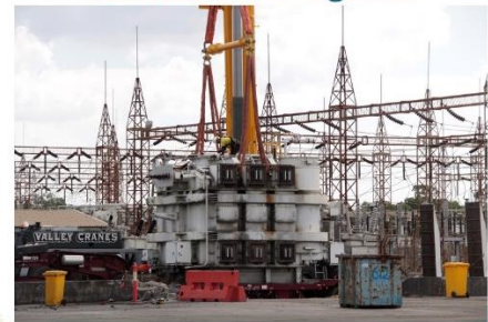
Line 1 Transformer Lid Removal (14/3/2019)
