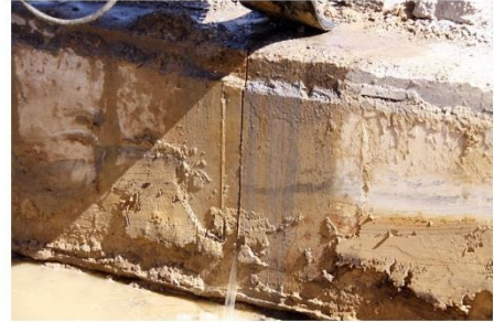
Saw cutting of Line 1 fume duct culvert (9/4/2019)
