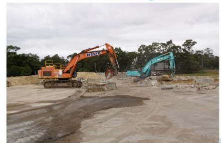
Removal of Line 1 foundations (4/4/2019)
