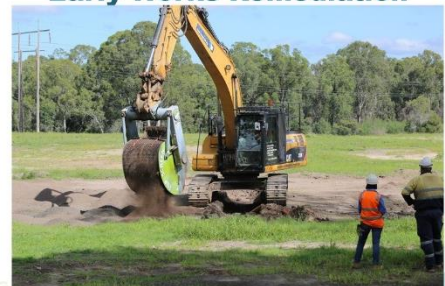
Flip Screen Trial at 2 Dawes Ave (11/4/2019) – successful but slow if material is wet.
