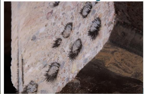
Magnetised reo in Line 1 (27/2/2019)
