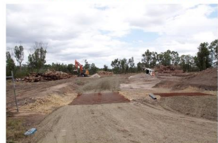
Rumble grids installed at Hart Rd Municipal Landfill (21/2/2019).
