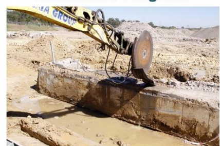
Saw cutting of Line 1 fume duct culvert (9/4/2019)
