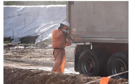
Wheel Washing at Early Works Stockpiling Area (22/3/2019)
