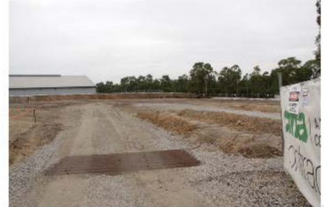
Early works stockpiling area with rumble grid in foreground (31/1/19)
