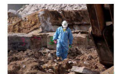
AECOM Site Auditor & Ramboll Visit - Inspection of ACM-Contaminated Line 3 Foundations (19/2/2019)
