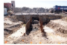
Stormwater drain on the west side of Line 3, 1500mm diameter & >1.5m deep (12/2/2019)
