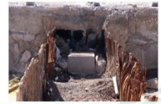
Stormwater drain on the west side of Line 3, 1500mm diameter & >1.5m deep (12/2/2019)
