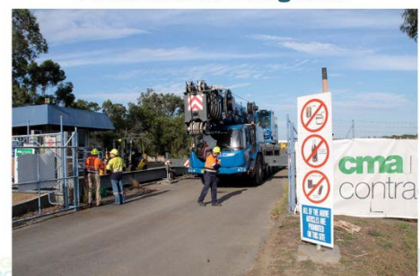
Mobile crane setting up to relocate the south weighbridge (22/1/2019)
