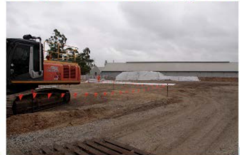
Geotextile being used to cover asbestos contaminated soils (1/2/2019)
