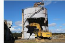
L3S alumina silo demolition in progress
