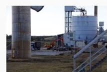
L3S scrubber tower felled and preparing to fell L3S alumina silo bucket elevator tower
