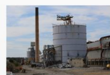
Demo of L3S alumina silo bucket elevator in progress
