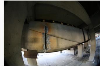
Line 3 cathode busbar after lancing. Cut to 5.7m lengths to fit a standard GP container. 100mm left at top will be cut by excavator during demolition.
