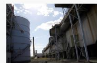
Separations made between L3S scrubber and L3 building in preparation for scrubber tower fell
