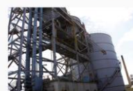
Separations made between L3S scrubber and L3 building in preparation for scrubber tower fell
