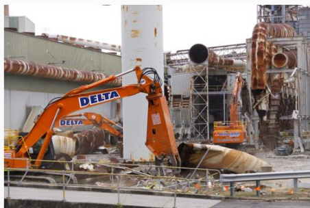
Demolition of Line 1 & 2 south dry scrubber fans and ductwork.
