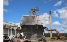
L3S alumina silo demolition in progress
