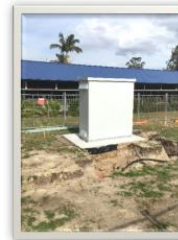
New 11kV switchboard
