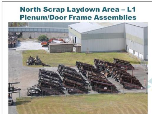
This is the North Scrap Lay Down Area for the steel scrap so they're all the Line 1 plenums and door frame assemblies. Plenums were used for removing pot fumes from pots to direct the gases to the scrubbing system. We're using an excavator with shears and grabs to process the scrap and load it into scrap trucks. Then they are taken down to Newcastle for recycling.
