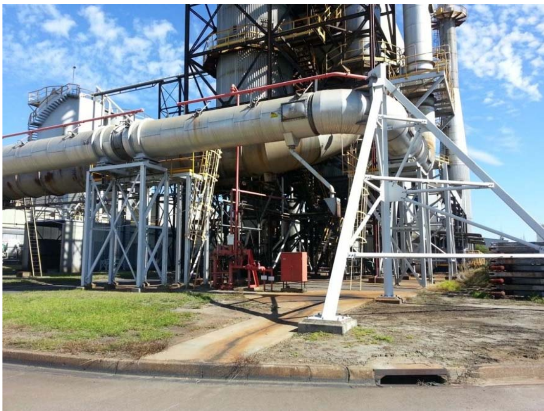
Plate 9: Bake Furnace Scrubber
