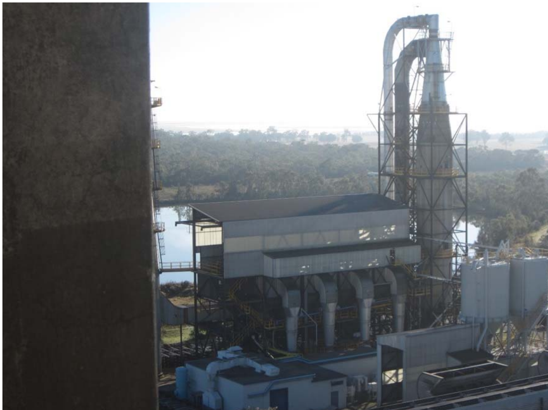
Plate 8: Bake Furnace Scrubber
