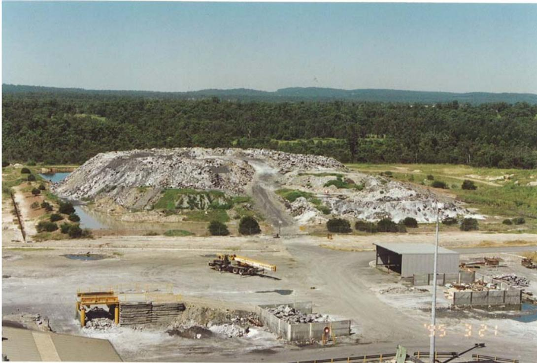
Figure 15 View of capped waste stockpile prior to capping (photo courtesy Hydro)
