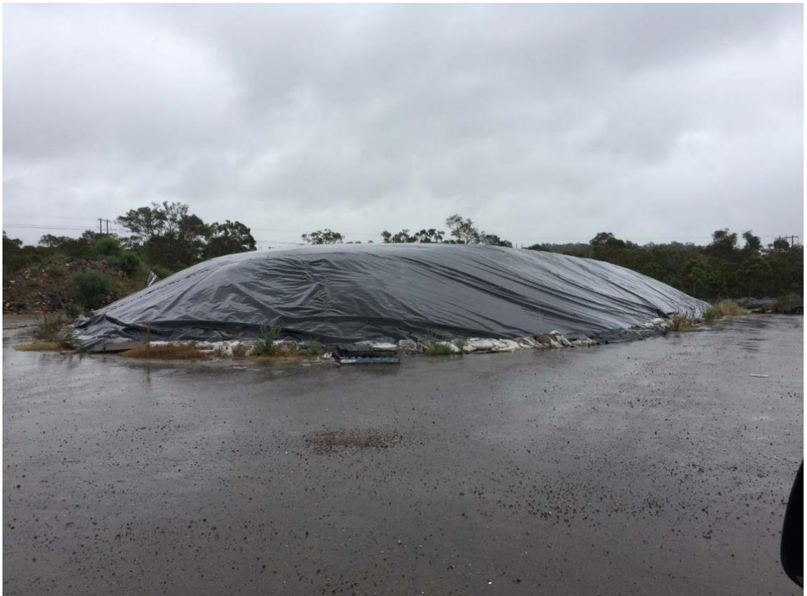
Figure 8 Typical External Stockpile – asbestos contaminated material
