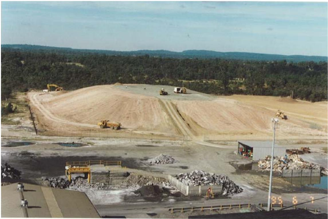
Figure 13 Construction of capping over capped waste stockpile (photo courtesy of Hydro)
