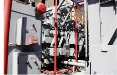
Wormalds are currently disconnecting the sprinklers to the Fuji rectifier units in preparation for demolition
