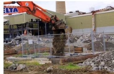
Backfilling of 17CS dump station void with clean soil stockpiled from the clay borrow pit remediation in 2015
