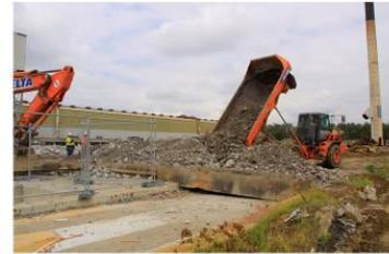
Backfilling of 17CS dump station void with pulverised concrete
