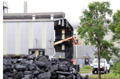
Removal of end wall of building 68C – anode storage area (to be used for storage of demolition waste)
