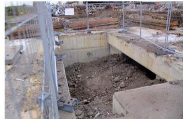
17CS dump station void partially filled
