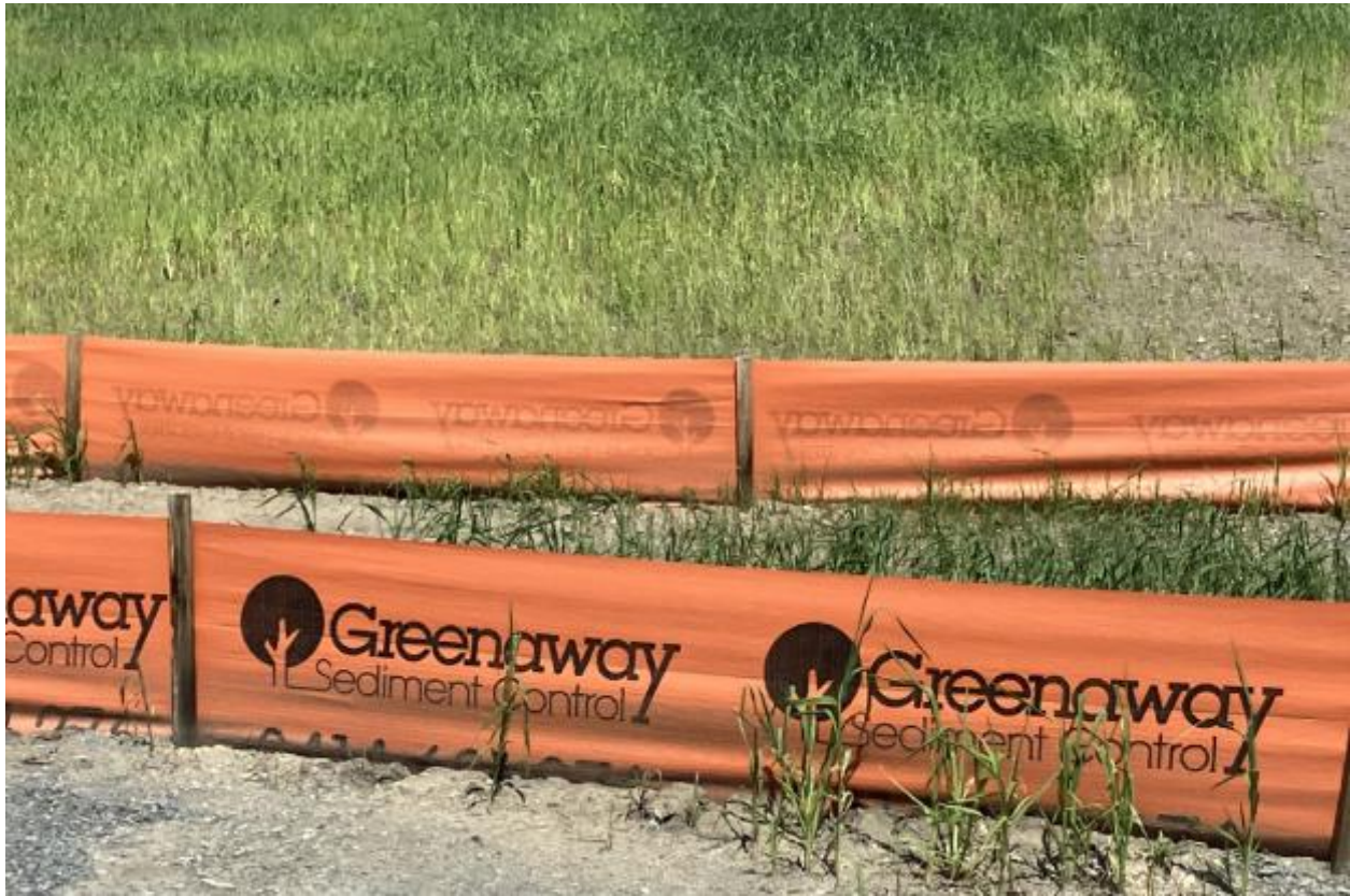
Temporary silt fencing in place until areas fully stabilised
