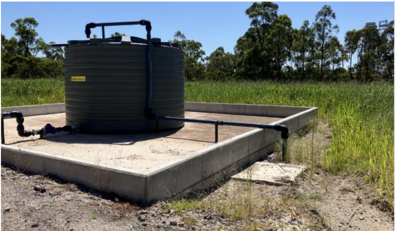
Area bunded with pit drain protection
