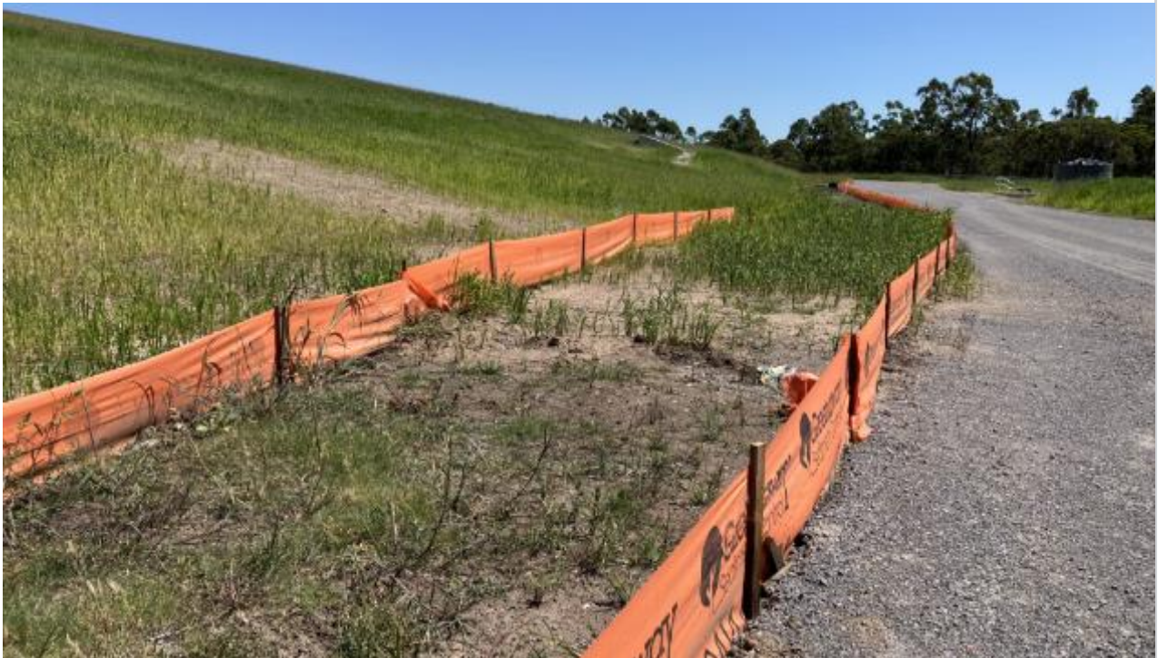
Double silt fencing around the perimeter of Containment Cell appeared in good condition.
