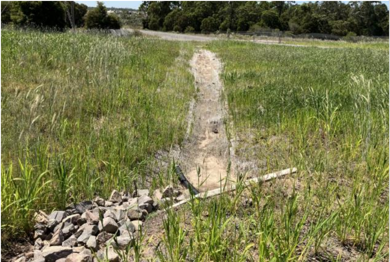
Rock placement and channel constructed to divert water into culvert
