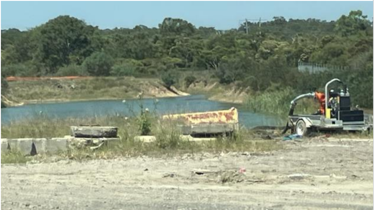
Dam onsite (known as the west surge pond) with pump for dewatering if required.
