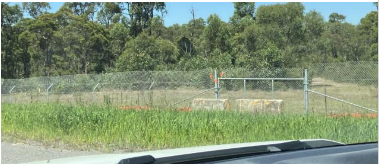
Silt fencing also installed along fauna fencing with plans to soon remove as the permanent grass starts to come in.
