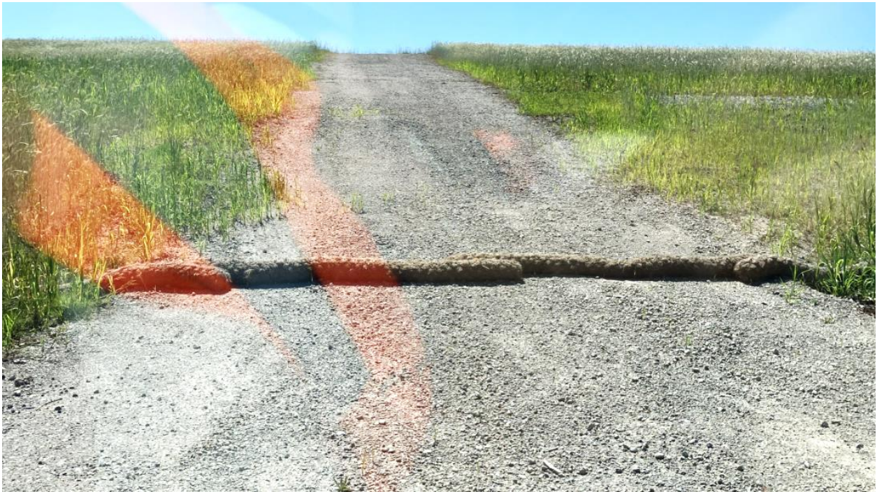
Access path to gas vent. Coir logs in place as an additional measure to manage high flow areas.
