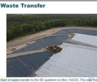
tart of waste transfer to the SE quadrant on Mon 13/2/23. This was the cementtabilised pond sediments from the west surge pond. An initial pad of 'fluffy' layer naterial was placed at 1.7m thick using a 36T digger.
