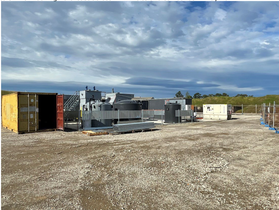
Photo 5: View looking northeast across WWTP site and surrounds in May 2022.
