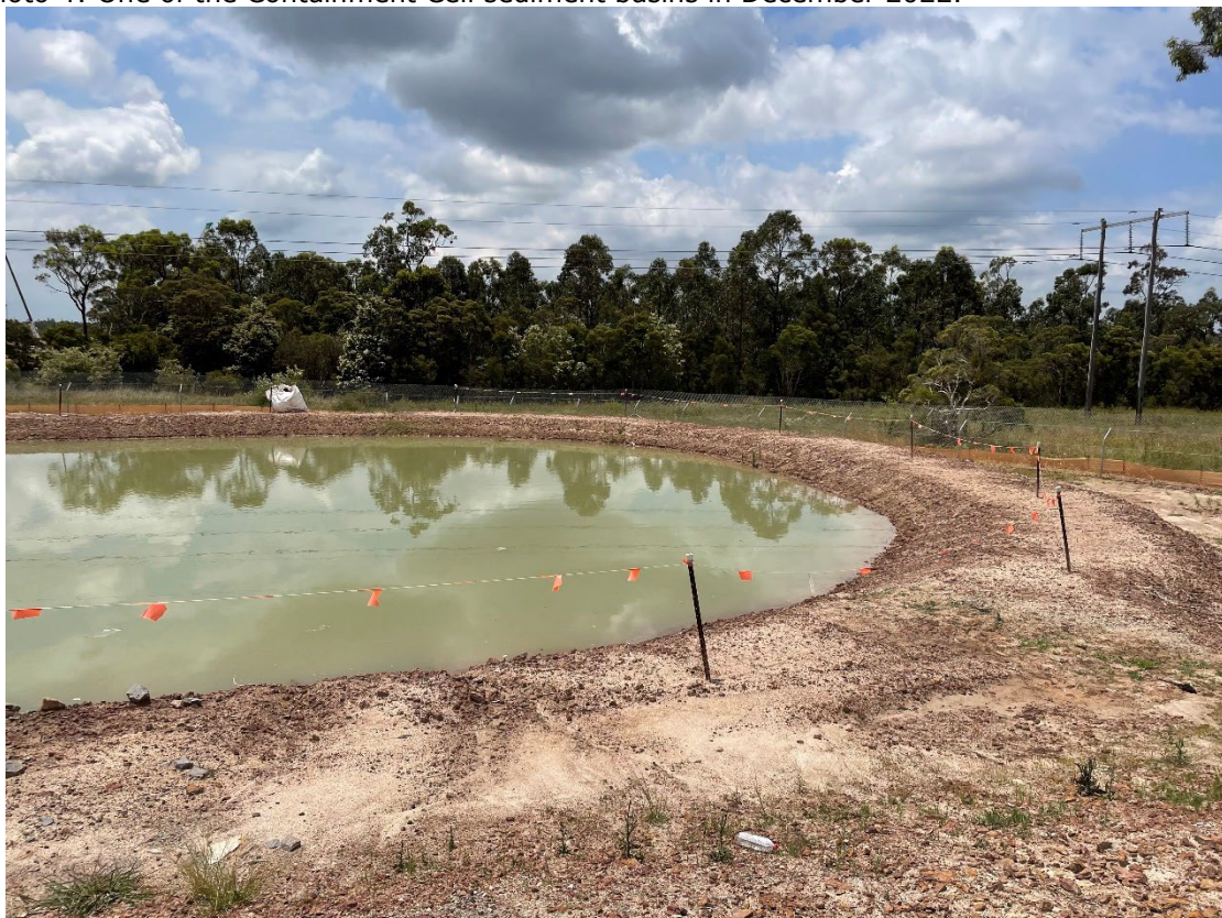
Photo 4: One of the Containment Cell sediment basins in December 2022.
