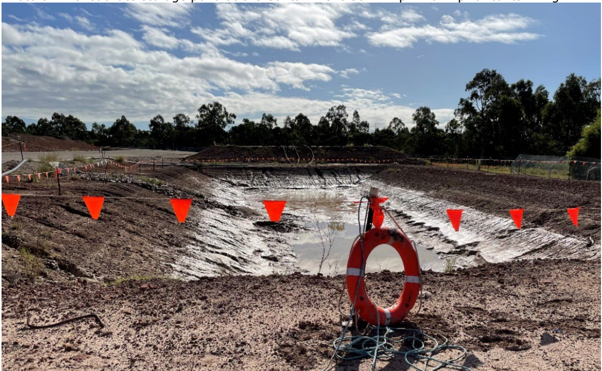
Photo 8: The leachate storage pond at the Containment Cell in April 2022 prior to its lining.
