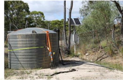
CREA PRO 24V solar powered bore pump and 10,000L leachate tank (15/2). FUT Leachate is now being transferred to the TWTP periodically.
