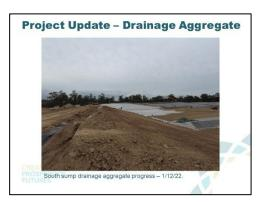
AW: This one is a bit later on, four days later. Southern sump is filling up. They just had to leave a small section where the big 450 diameter riser pipes get installed and you can see a gap there on the batter. There's a gap in the soil confining layer, and that's where those pipes are going to go. We'll see later on.
