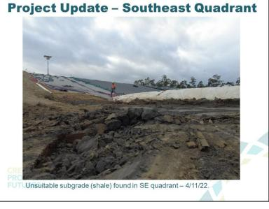
AW: That's as close up of the shale that we found, which is very crumbly rock and the specification from GHD calls for the subgrade to be firm and unyielding, and the shale is a very soft, crumbly rock, so it's not suitable, so it had to be removed, ripped out and replaced and then recompacted.
