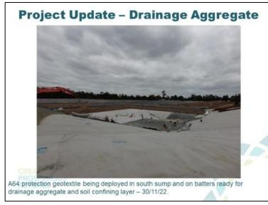
AW: The same thing, protection geotextile is being put on the batters and starting to be put into the sump. So it's there to protect the liner from the drainage aggregate that's being placed in the sump and also protects the side walls when you're placing the clay for the soil confining layer.
