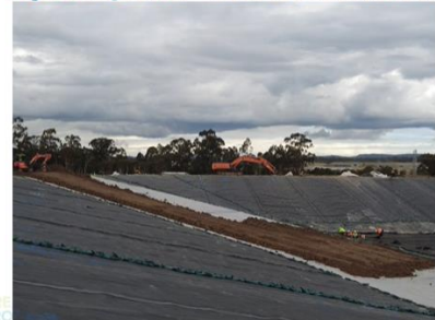
NE ramp soil confining layer and GCD installation in north sump – 6/9/22
