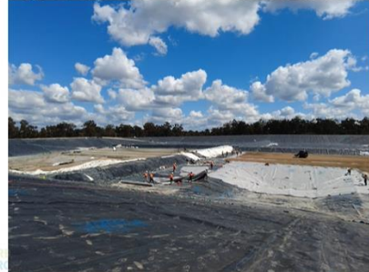
Protection geotextile deployment in the NE quadrant – 20/9/22.
