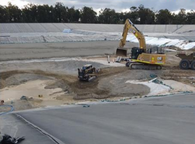
CRG PRO FLU South sump cleanout of gravel and sand - 13/9/22
