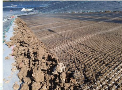
NE ramp soil confining layer and geonet – 7/9/22.
