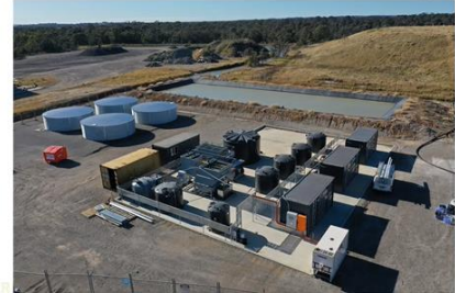
Temporary Water Treatment Plant – process commissioning is underway.
