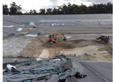
CRG PRO FLU South sump cleanout of gravel and sand – 7/9/22
