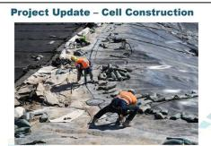
Secondary HDPE liner patch being extrusion welded to the existing secondary liner – 17/8/22. Small circles are patches at the T joints. Large
