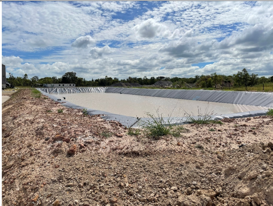
Photo 7: The Leachate Storage Pond adjacent to the TWTP. Note that the pond contains rainwater at the time of this photo (following significant rainfall in January 2022)
