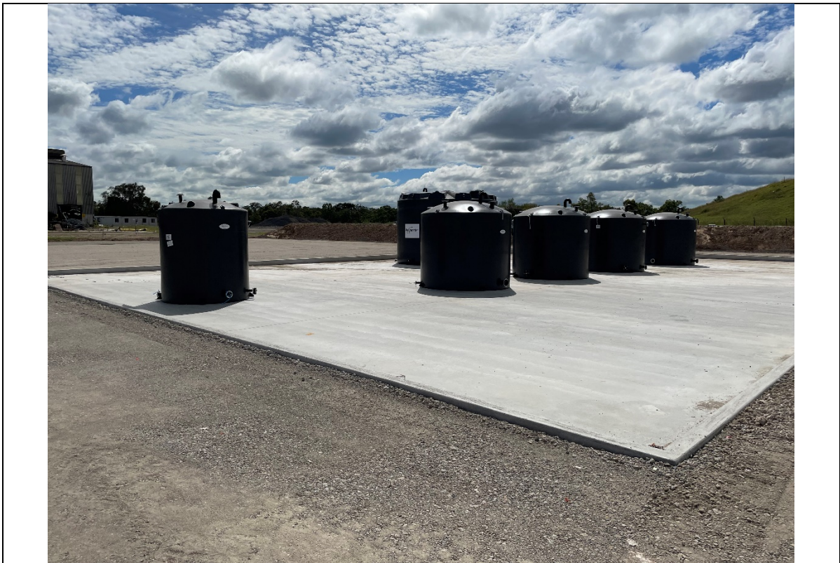
Photo 6: The concrete pad and bund for the TWTP, with some of the tanks for the plant delivered awaiting installation
