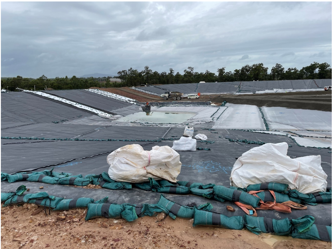
Photo 2: View over the southern end of the Containment Cell in February 2022
