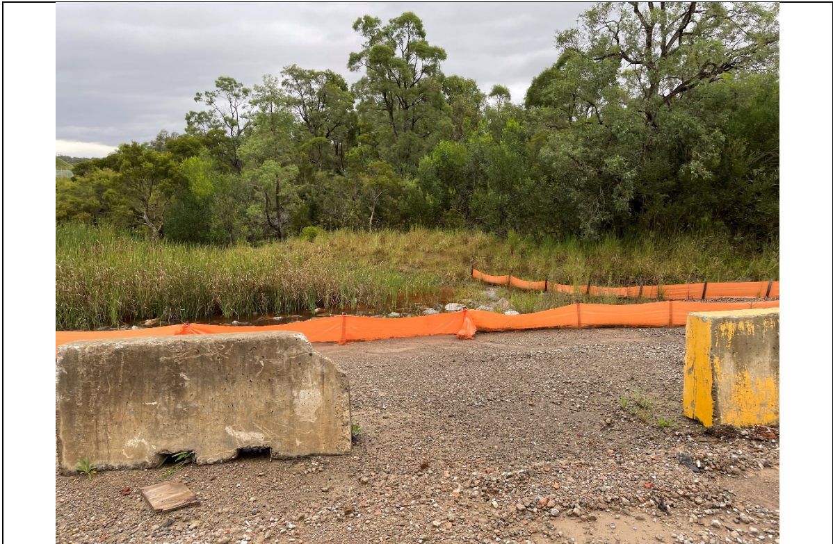
Photo 5: Example of the sediment fencing installed along the haul road
