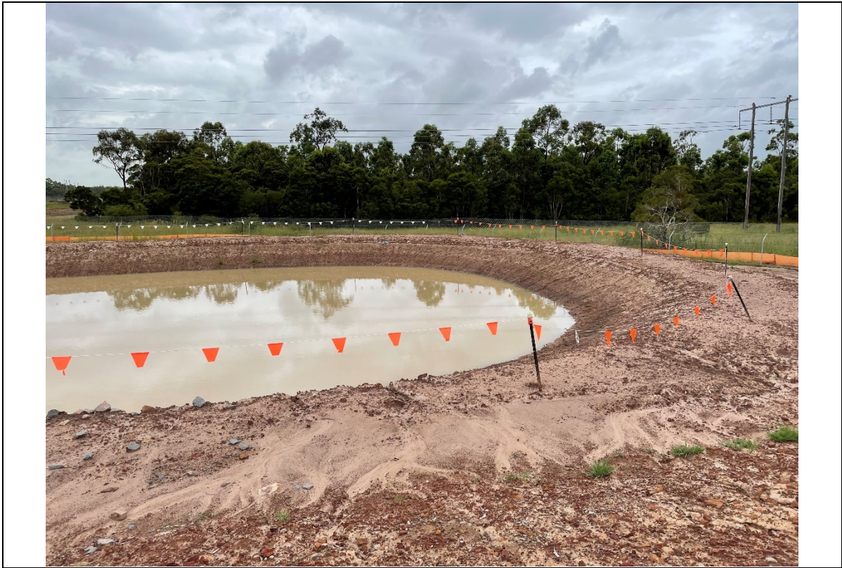
Photo 3: One of the Containment Cell sediment basins in February 2022, after significant rainfall
