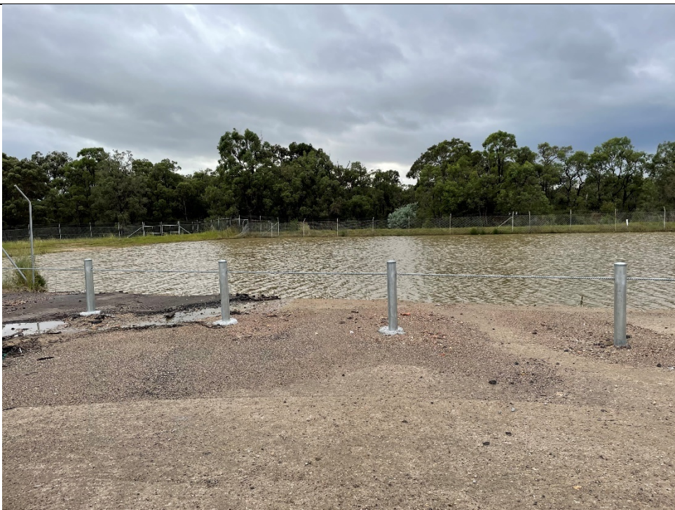
Photo 8: The Eastern Surge Pond in March 2022 following removal of sediments from the pond floor. The water level is indicative of the significant rainfall at the site over summer of 2021/2022.
