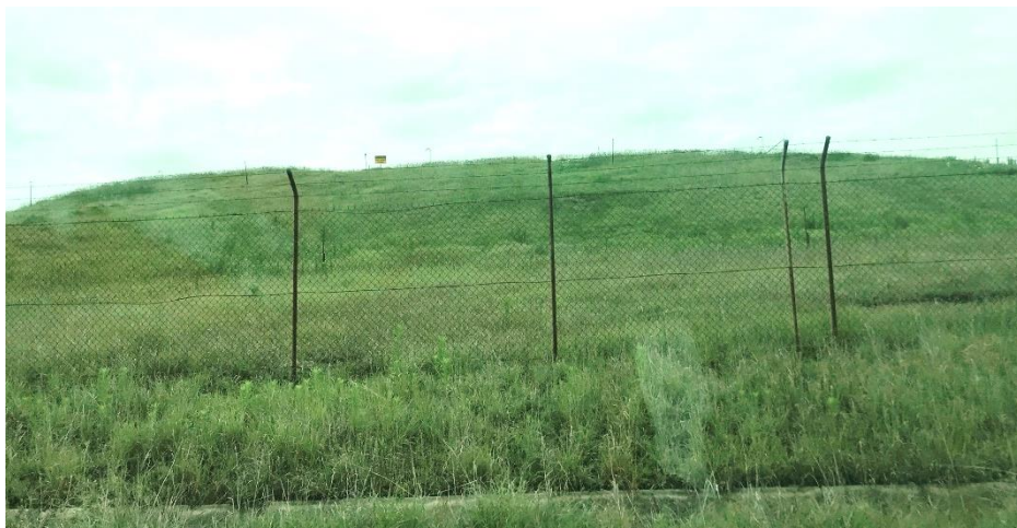
Photo 7 – Fencing at Capped Waste Stockpile
