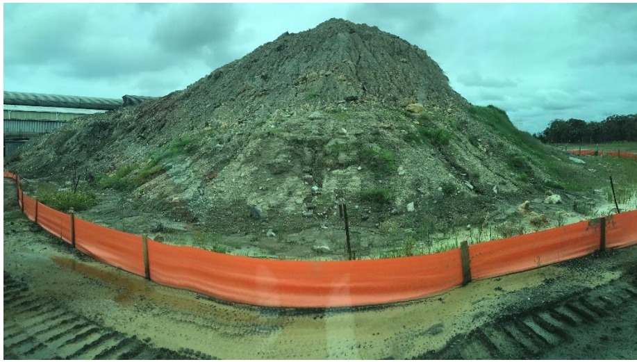
Photo 21 – Stockpile with Erosion and Sediment Controls
