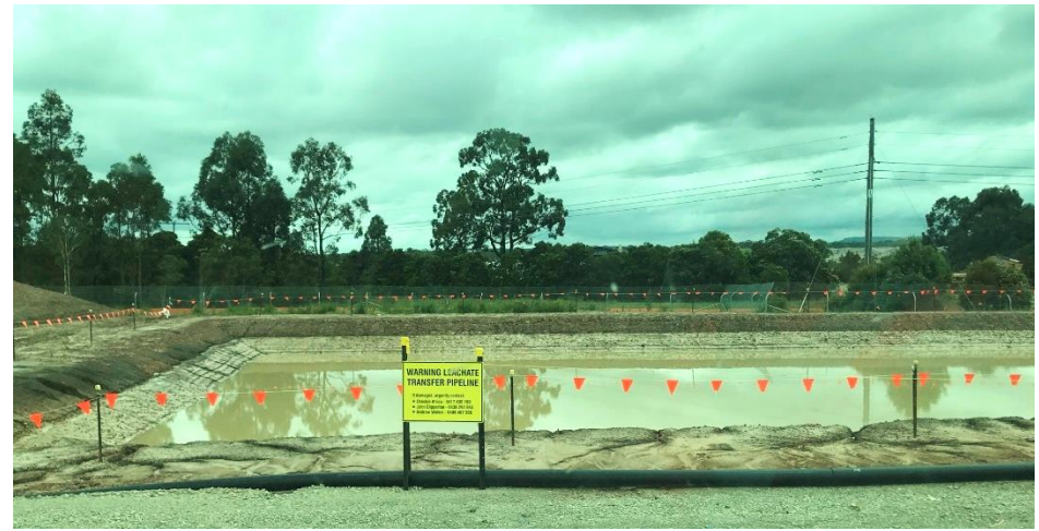
Photo 25 – Newly constructed Sediment Basin at ECC with depth marker and safety ring.
