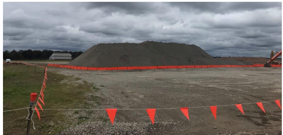
Photo 24 – Stockpile of imported sand for the leak detection layer in the Containment Cell with Erosion and Sediment Controls and work boundary flagging.
