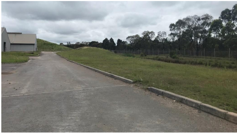
Photo 9 – Shed haul route
