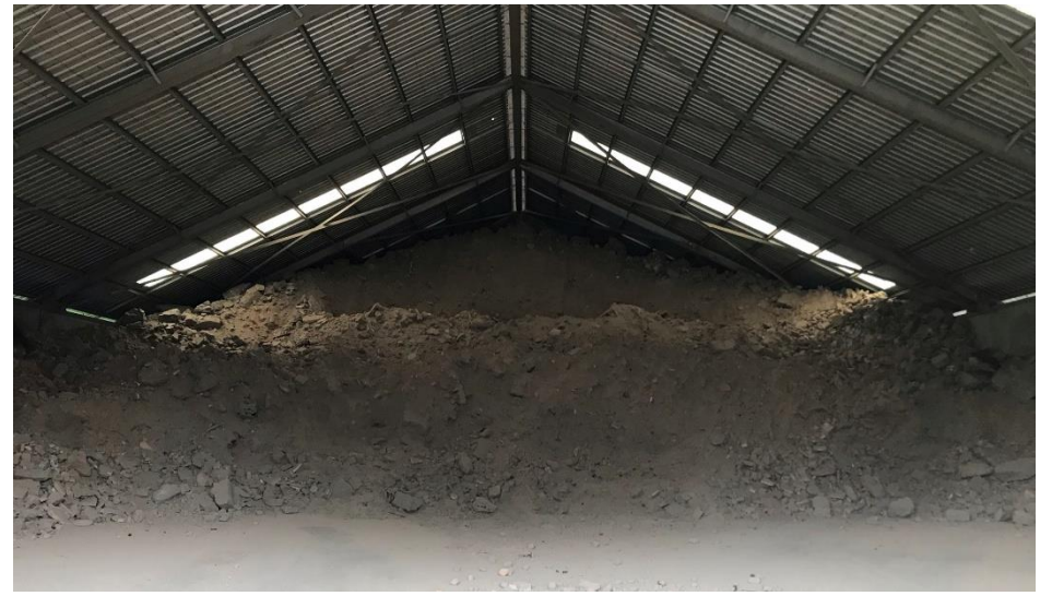
Photo 14 – Interior of waste containment shed
