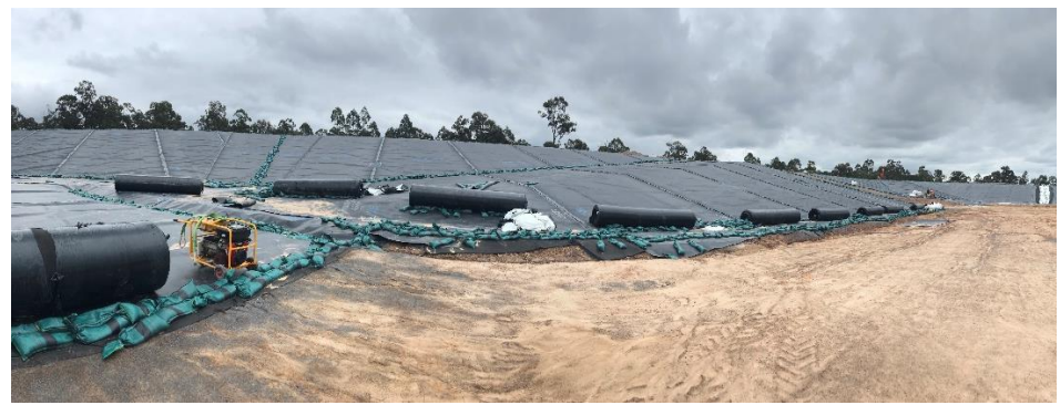
Photo 30 – Containment Cell with geosynthetic lining - northern batter
