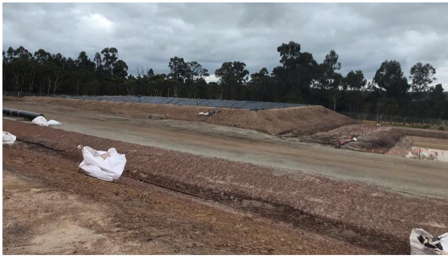
Photo 35 – Leachate Pond adjacent to Containment Cell
