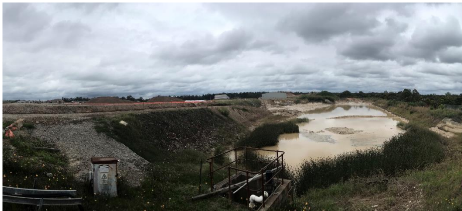
Photo 39 – Remediation of the former smelter West Surge pond was ongoing.
