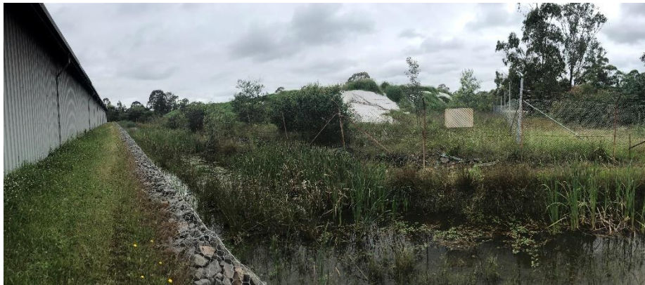
Photo 5 – Watercourse alongside site boundary with gabion wall
