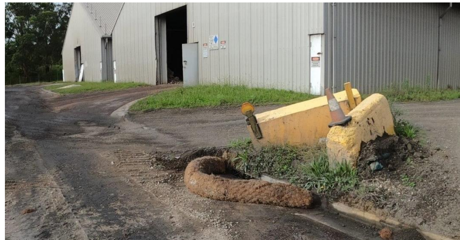
Photo 1B: Pit drain cleaned and coir logs established. CLOSED.
