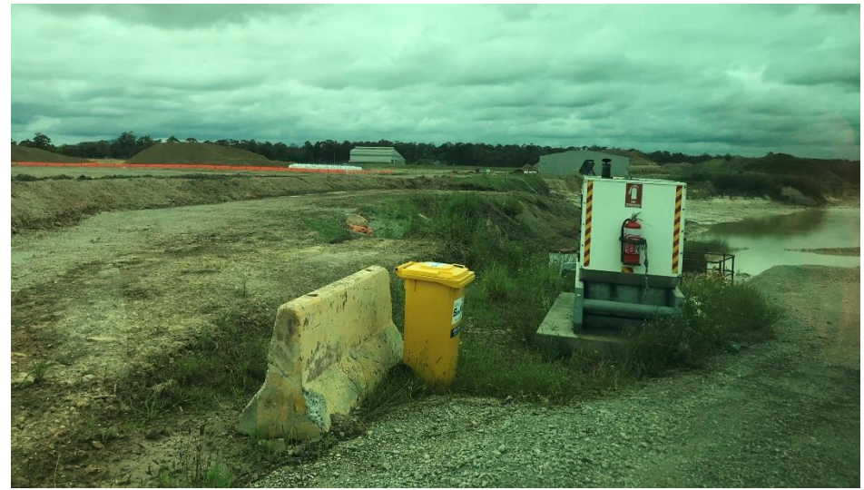
Photo 38 – Spill kit and fire extinguisher placed near the pump and generator at the former smelter West Surge Pond which was undergoing remediation.
