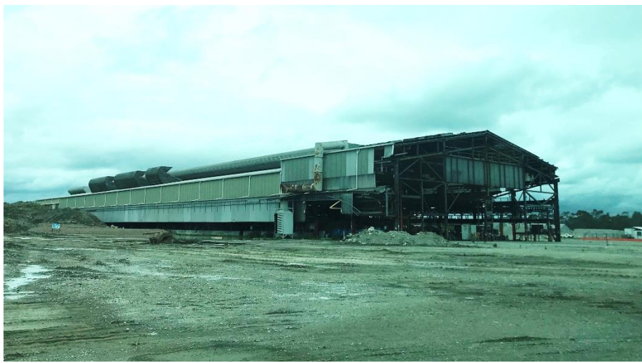
Photo 17 – Existing shed used for non-contaminated process waste storage
