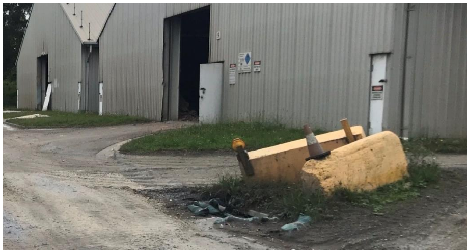
Photo 1A: Recommendation to maintain pit drains and use coir logs in place of sandbags
