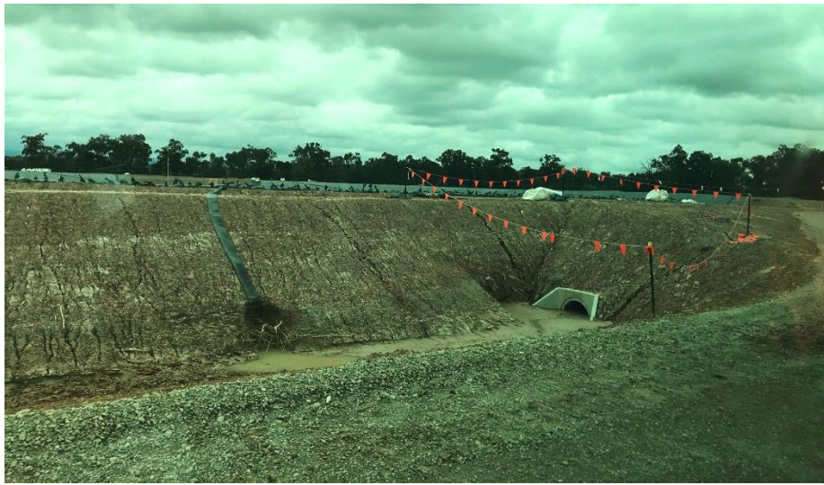
Photo 37 – Containment Cell - Erosion and sediment controls in place – Culvert 04 at the northeast ramp into the cell
