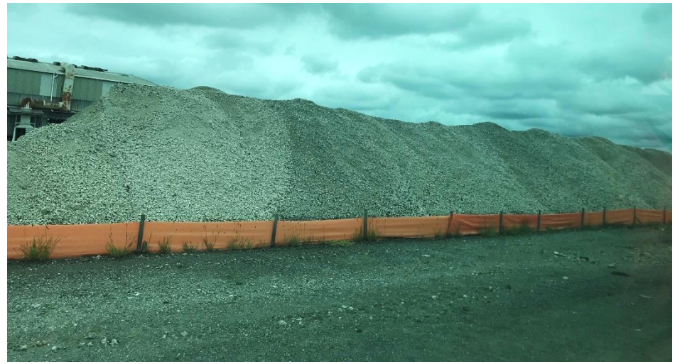
Photo 22 – Stockpile of crushed concrete with Erosion and Sediment Controls
