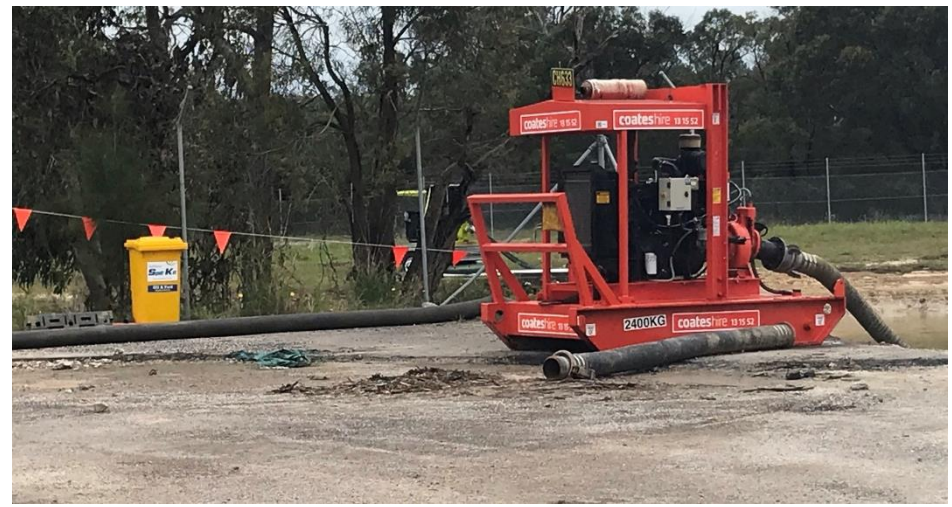
Photo 28 – Spill kit and pump generator at the East Surge Pond
