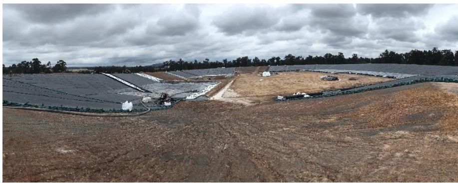
Photo 29 – Containment Cell with geosynthetic lining looking south
