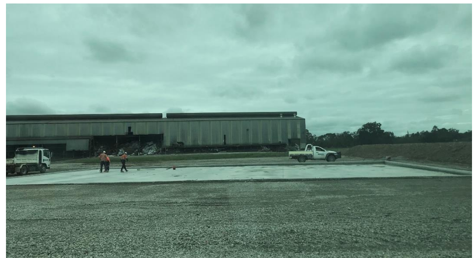
Photo 18 – Temporary Water Treatment Plant (TWTP) - construction of the bunding commenced.
