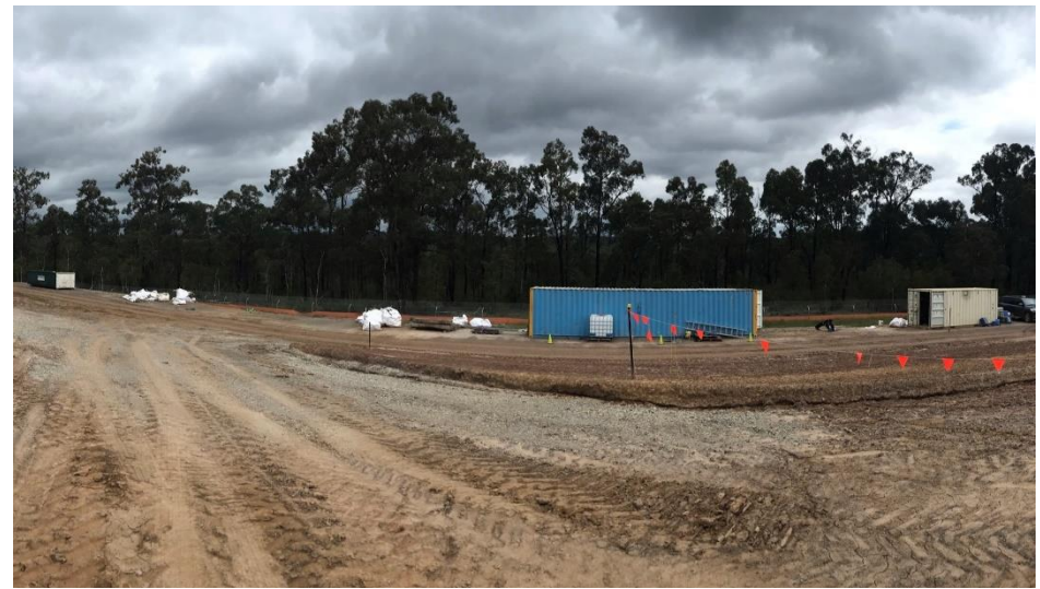
Photo 36 – Perimeter Road surrounding Containment Cell
