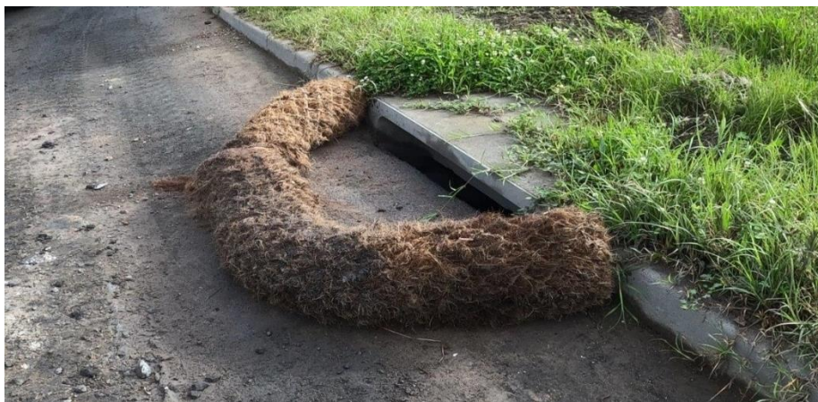
Additional coir logs have been put in place.
