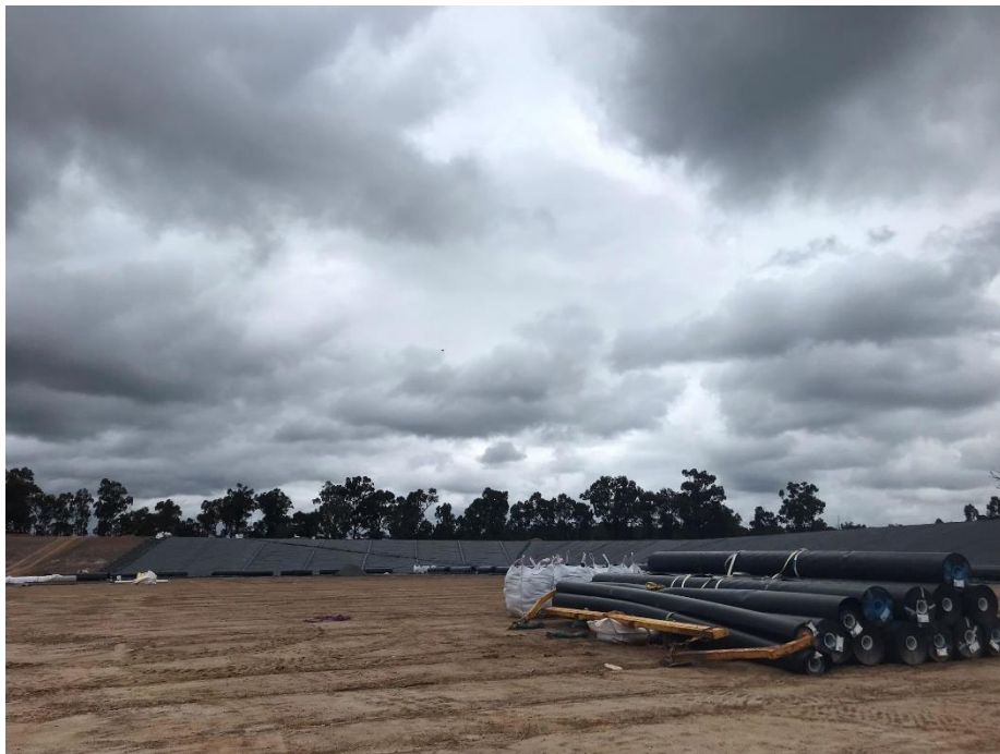
Photo 31 – Containment Cell looking towards the southern batter
