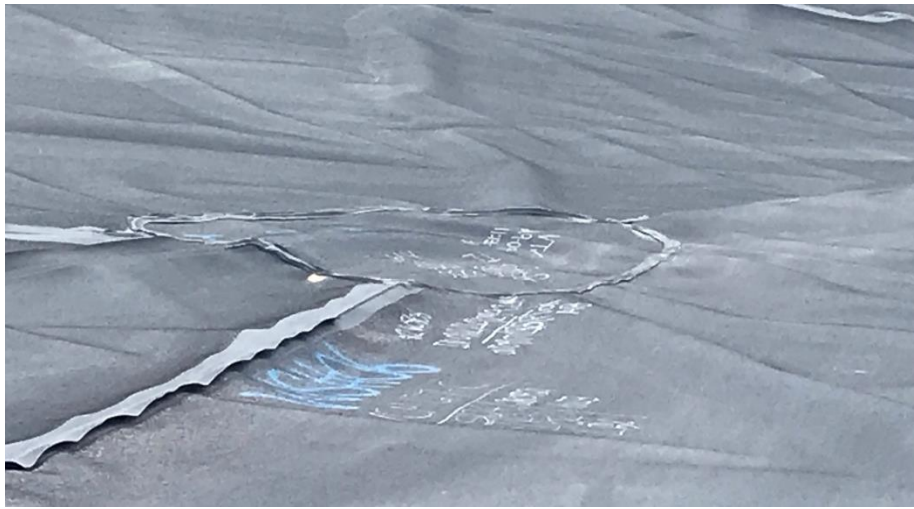
Photo 33 – Containment Cell testing marks
