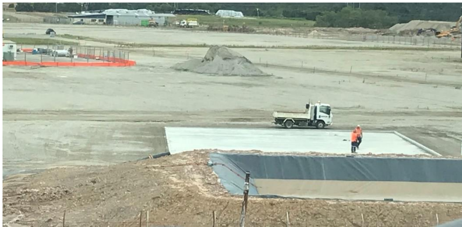
Photo 19 – Leachate Pond lined and operating, adjacent to TWTP to be used for collecting leachate from the Capped Waste Stockpile.
