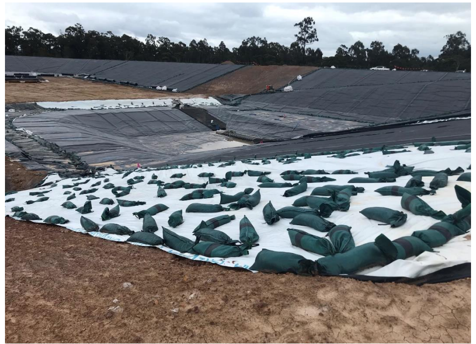
Photo 32 – Containment Cell – northern sump and northern batter
