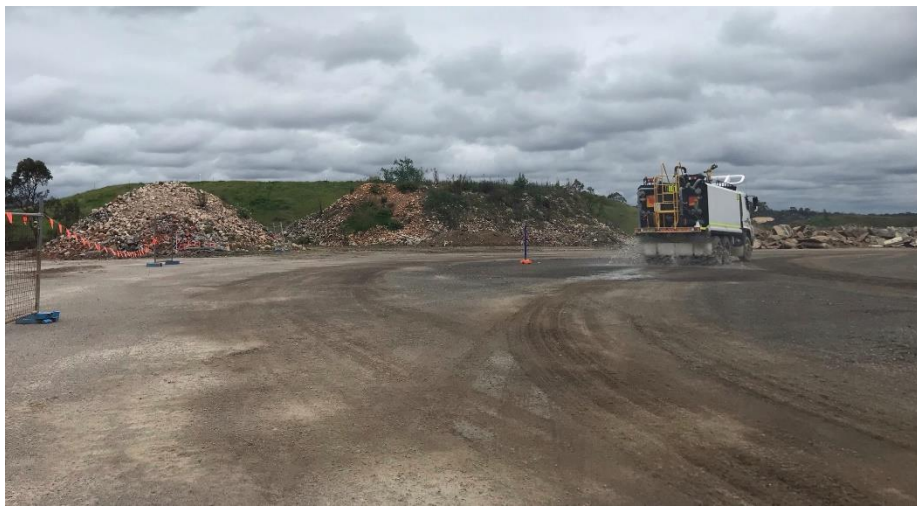
Photo 27 – Water Cart in operation near the East Surge Pond
