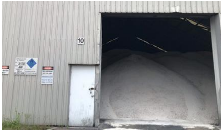
Photo 13 – Shed 10 stored with Gypsum
