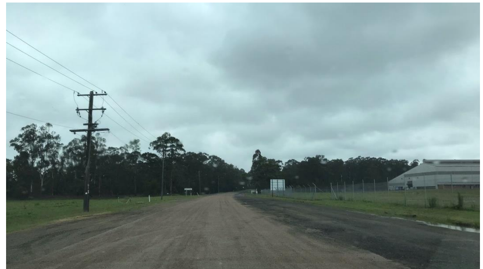
Photo 44 – Hart Road – no mud tracking or dust
