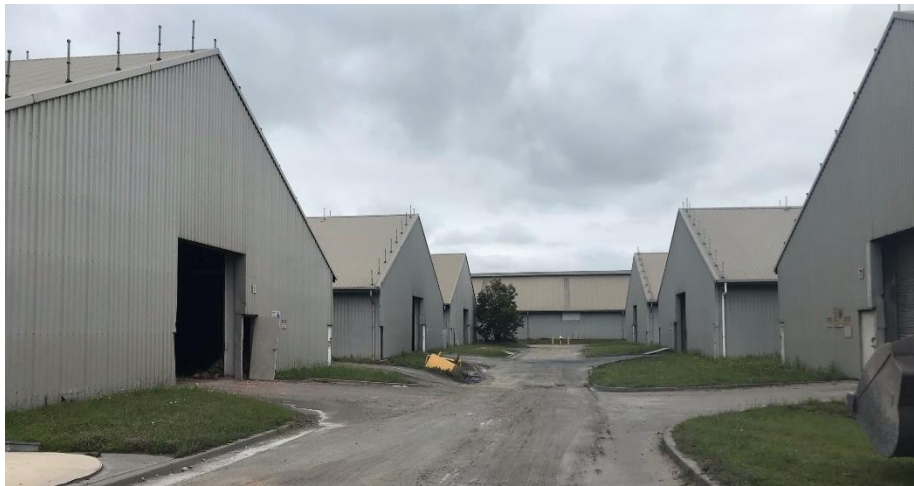
Photo 11 – Containment Shed area. Sheds 5, 6 and 9 contain Spent Potlining (SPL).
