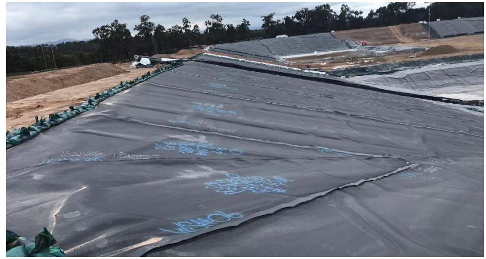
Photo 34 – Containment Cell testing marks
