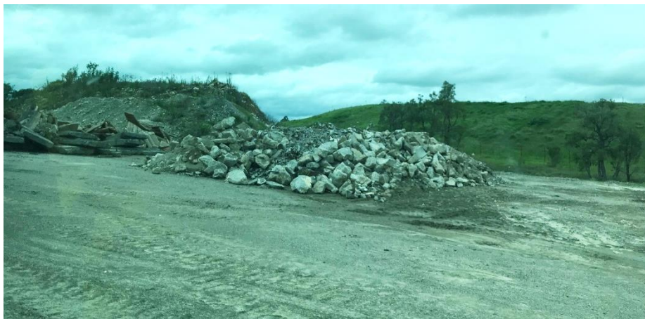
Photo 23 – Stockpile of Recyclable Concrete will be crushed and reused
