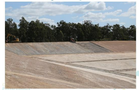
ECC Works – subgrade preparation on western batter (8/9/21)
