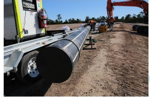
Butt welding of HDPE pipes. End cap installed (6/9/21)
