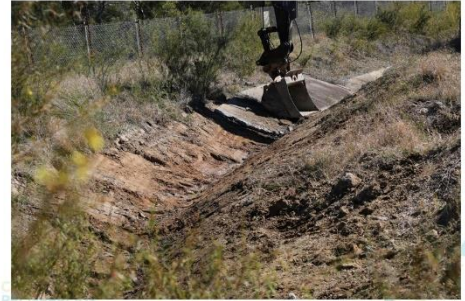
West Surge Pond – vee drain remediation (23/9/21)
