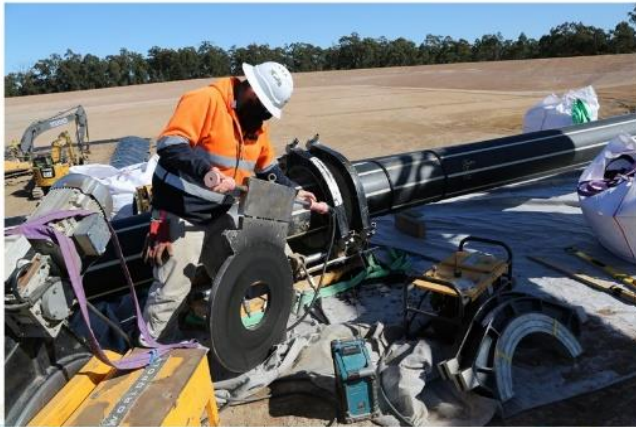
Heating platen for butt welding of HDPE pipes (6/9/21)
