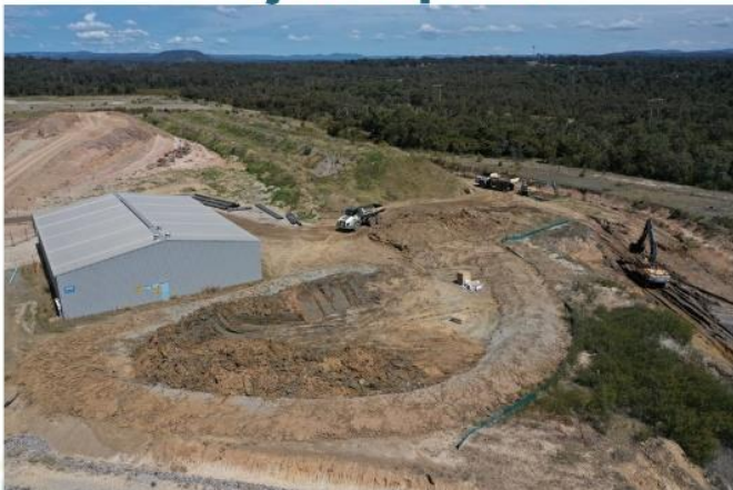
West Surge Pond – cement mixing bay #1 (28/9/21)
