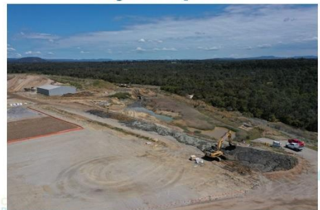
West Surge Pond – mixing bay #2 adding 4% cement (28/9/21)
