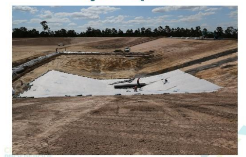
South sump – groundwater riser pipes installed (8/9/21)
