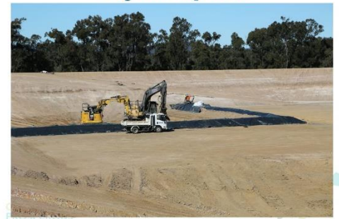
ECC Works – temporary stormwater bunds at south sump (6/9/21)
