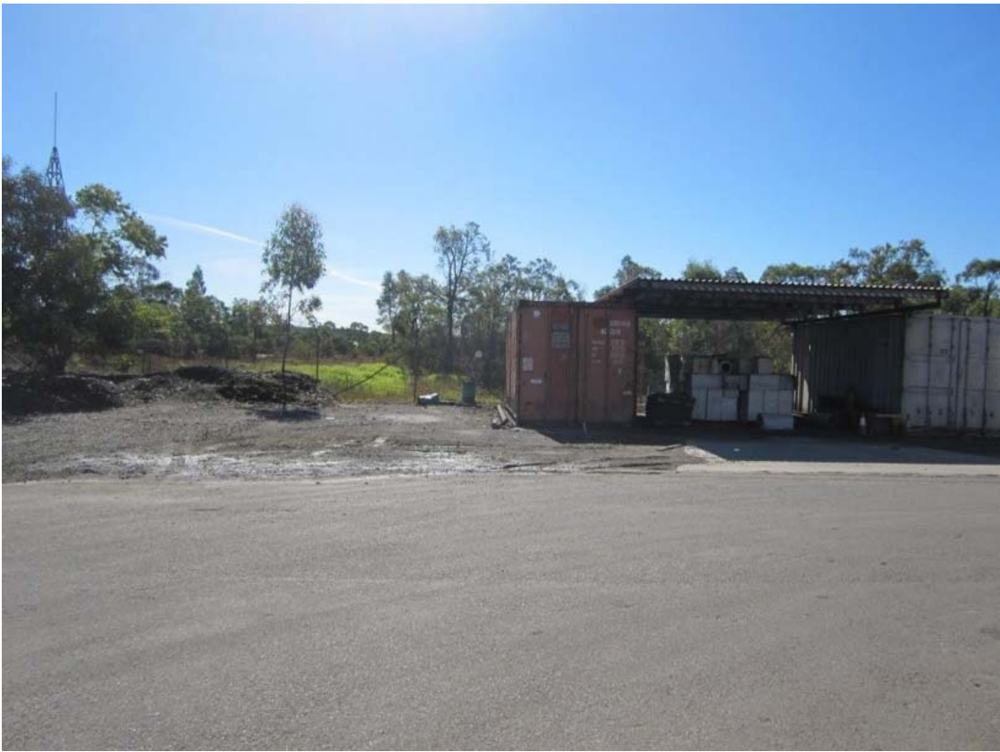
Plate 3: Diesel Spray Area
