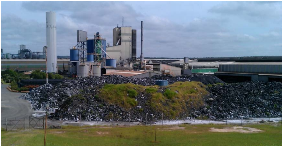
Plate 2: Anode Waste Pile
