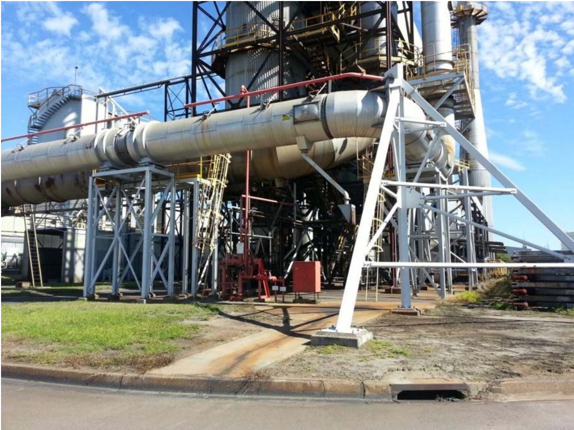
Plate 9: Bake Furnace Scrubber
