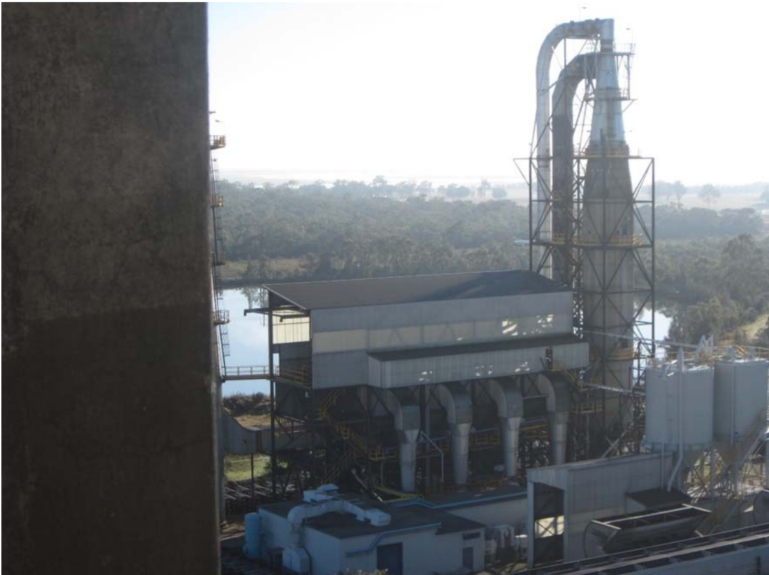
Plate 8: Bake Furnace Scrubber
