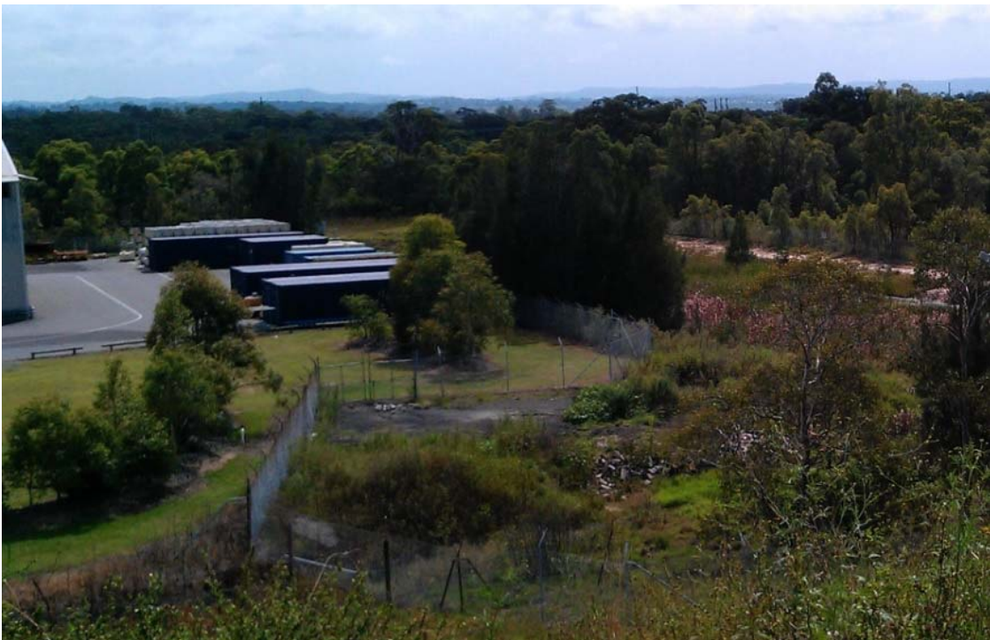
Plate 4: Drainage Lines near Capped Waste Stockpile and Anode Waste Pile
