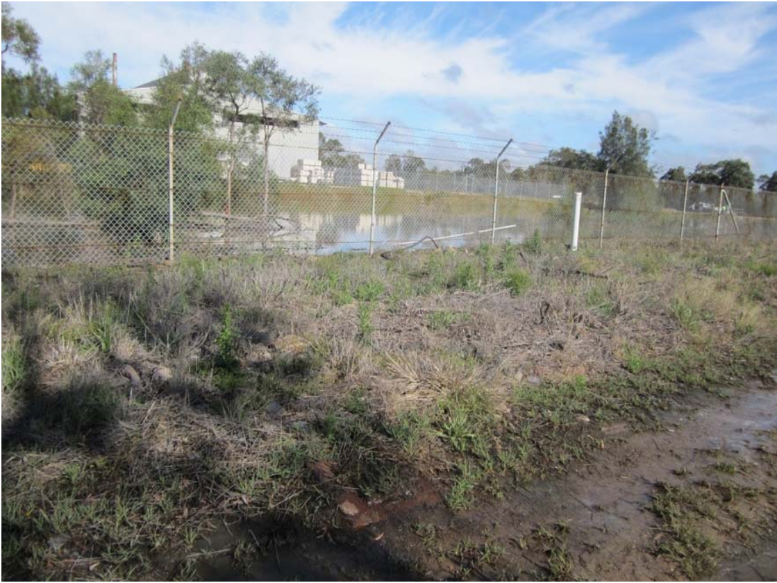
Plate 5: East Surge Pond
