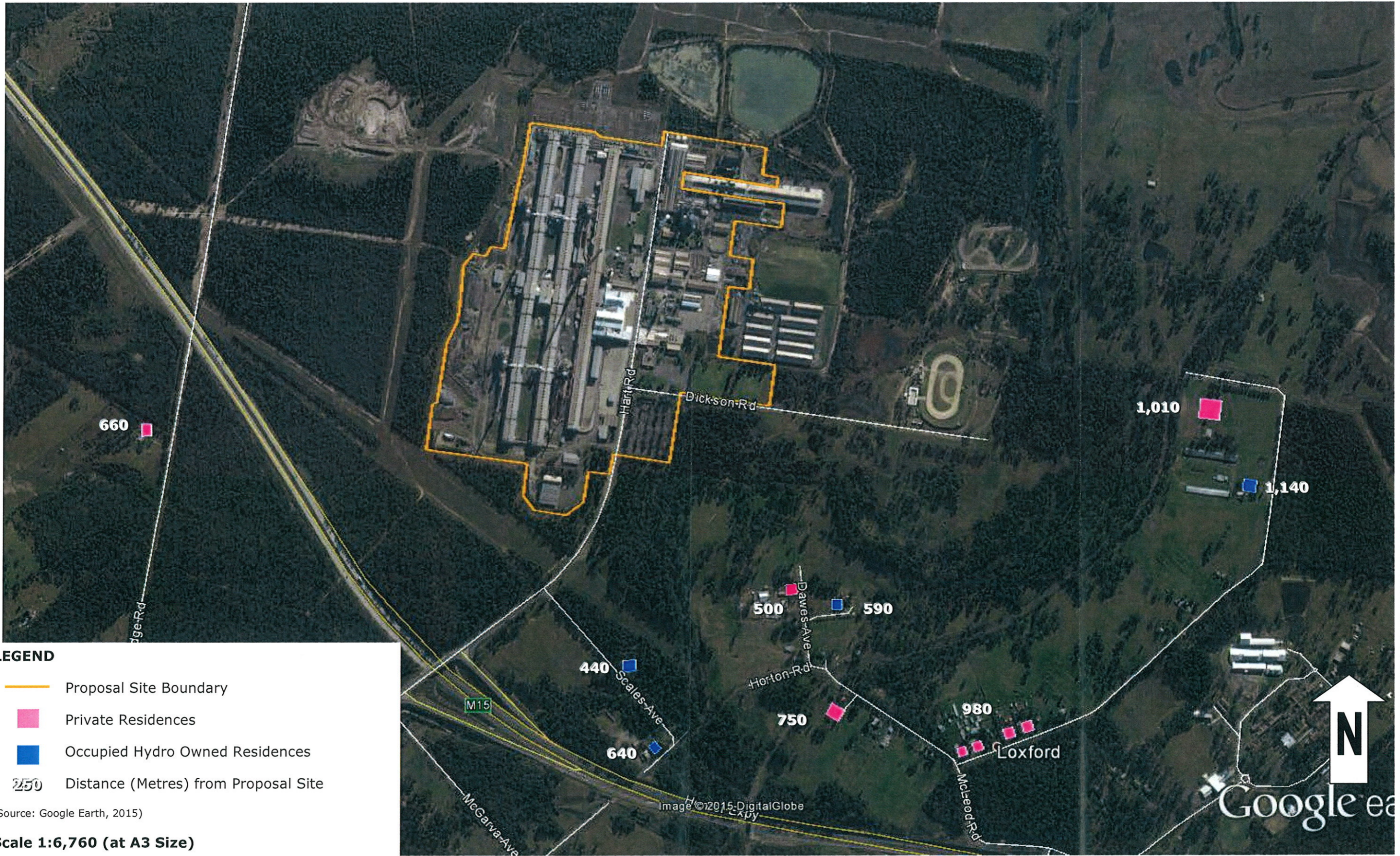
Hydro Aluminium Kurri Kurri: Stage 1 of the Demolition of the Former Aluminium Smelter at Kurri Kurri
