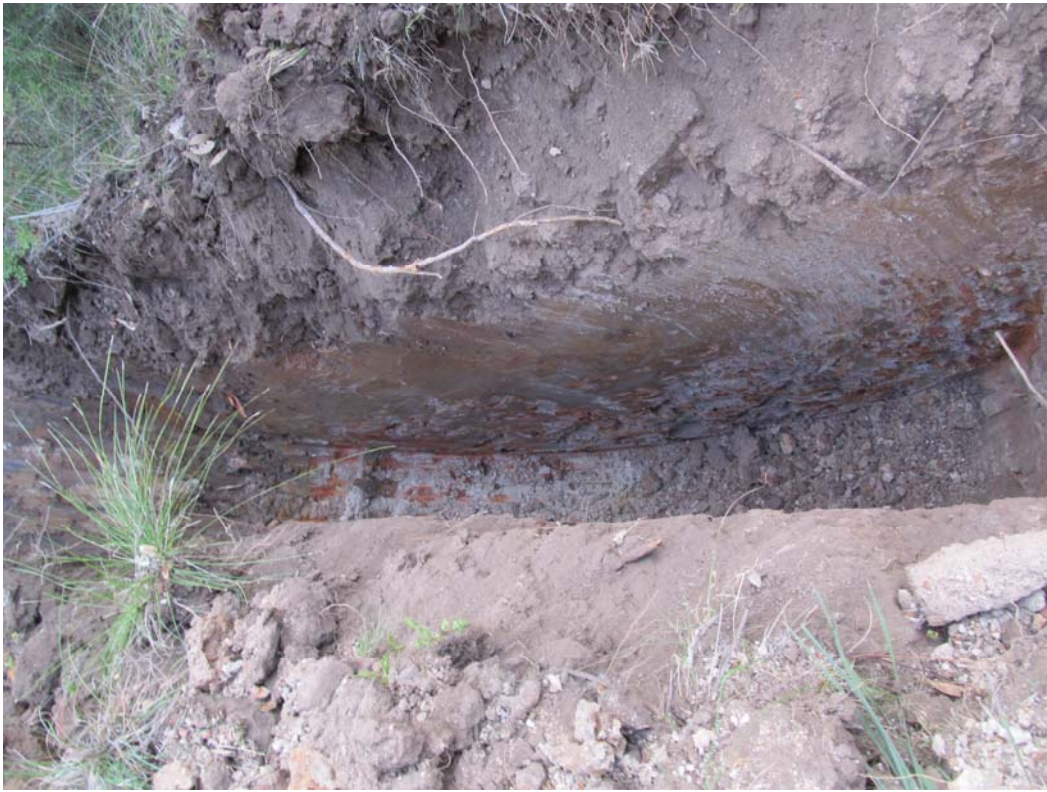
Photograph 8 Test Pit TP108
