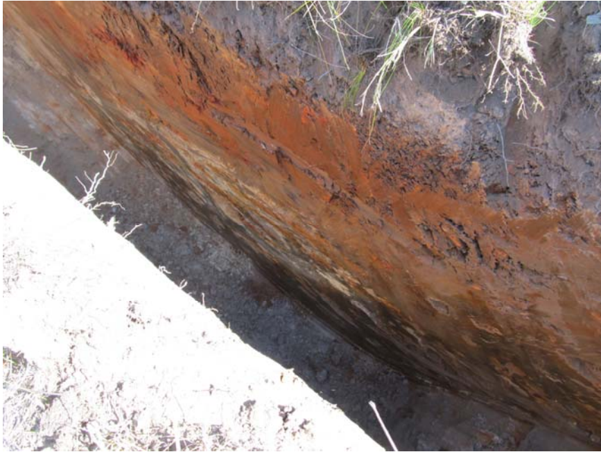
Photograph 3 Test Pit TP103
