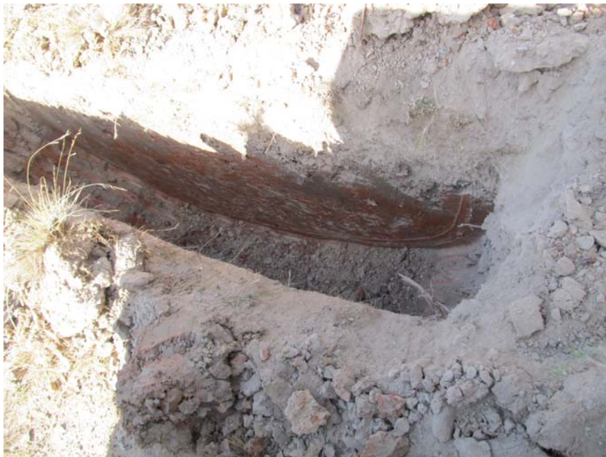
Photograph 4 Test Pit TP104
