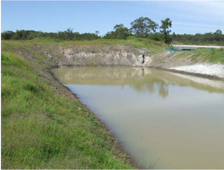
Photo 2 Sedimentation pond from Hunter Expressway works showing clayey soils in exposed banks in south-west of the Lumby Lane site
