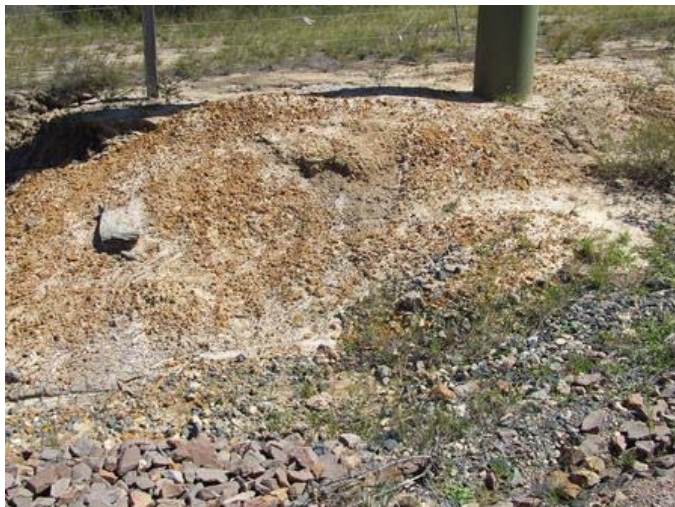
Photo 4 Showing clayey soils in rain washout at base of Energy Australia pole on Bishops Bridge Road
