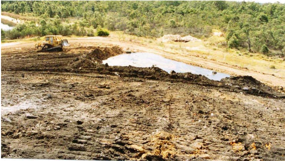
Plate 2: Showing water at the north east corner of the Alcan Mound during capping.
