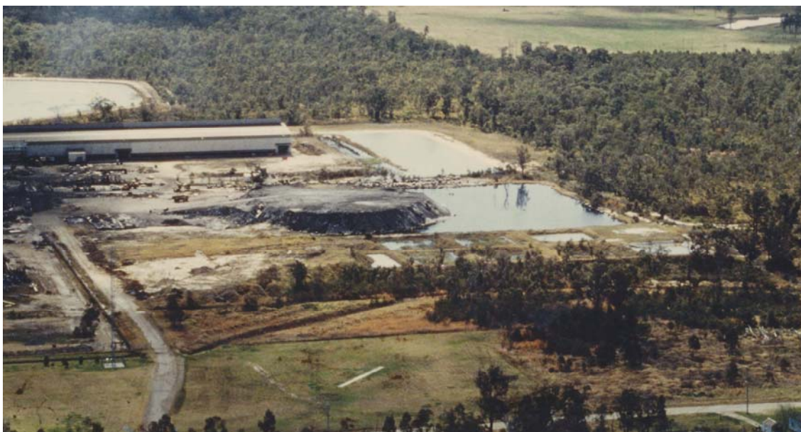
Plate 1: Showing water within the bund walls during capping, also shows the size of the East Surge Pond at the rear of the Alcan Mound.
