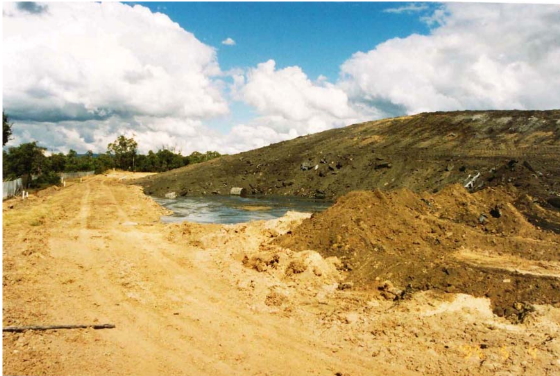
Plate 3: Showing water at the north east corner of the Alcan Mound during capping.
